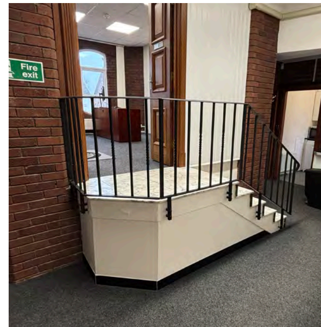
Stone clad stair and solid timber doors on first floor
