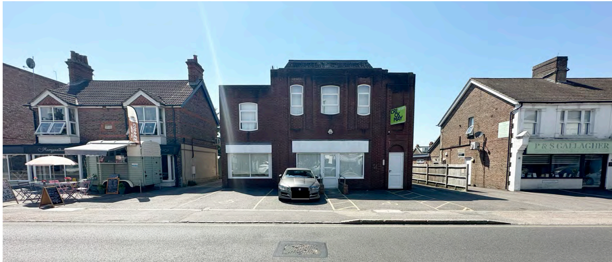
Site photo looking west across Sussex Road towards the existing building
