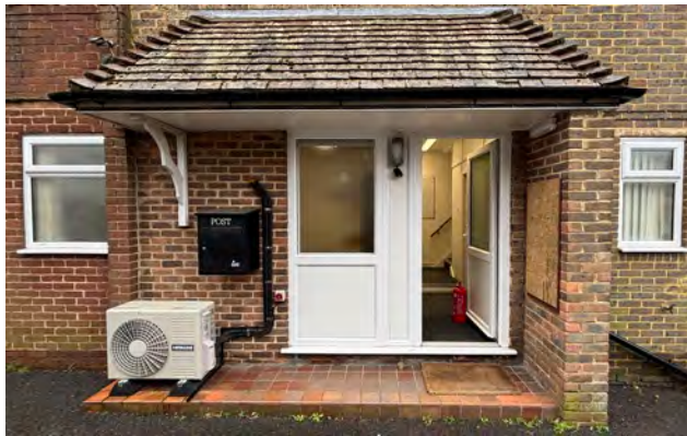
Side entrance with stepped access and hipped roof canopy with concrete tiles.
