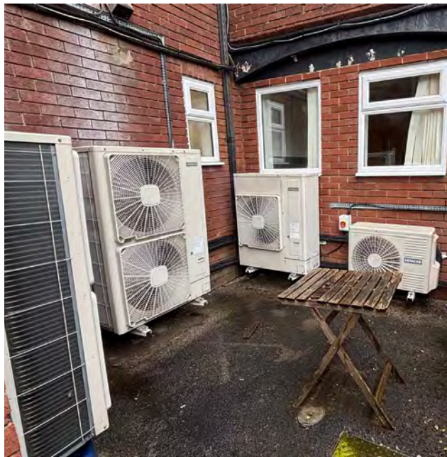
Gated external plant area to the south of the building
