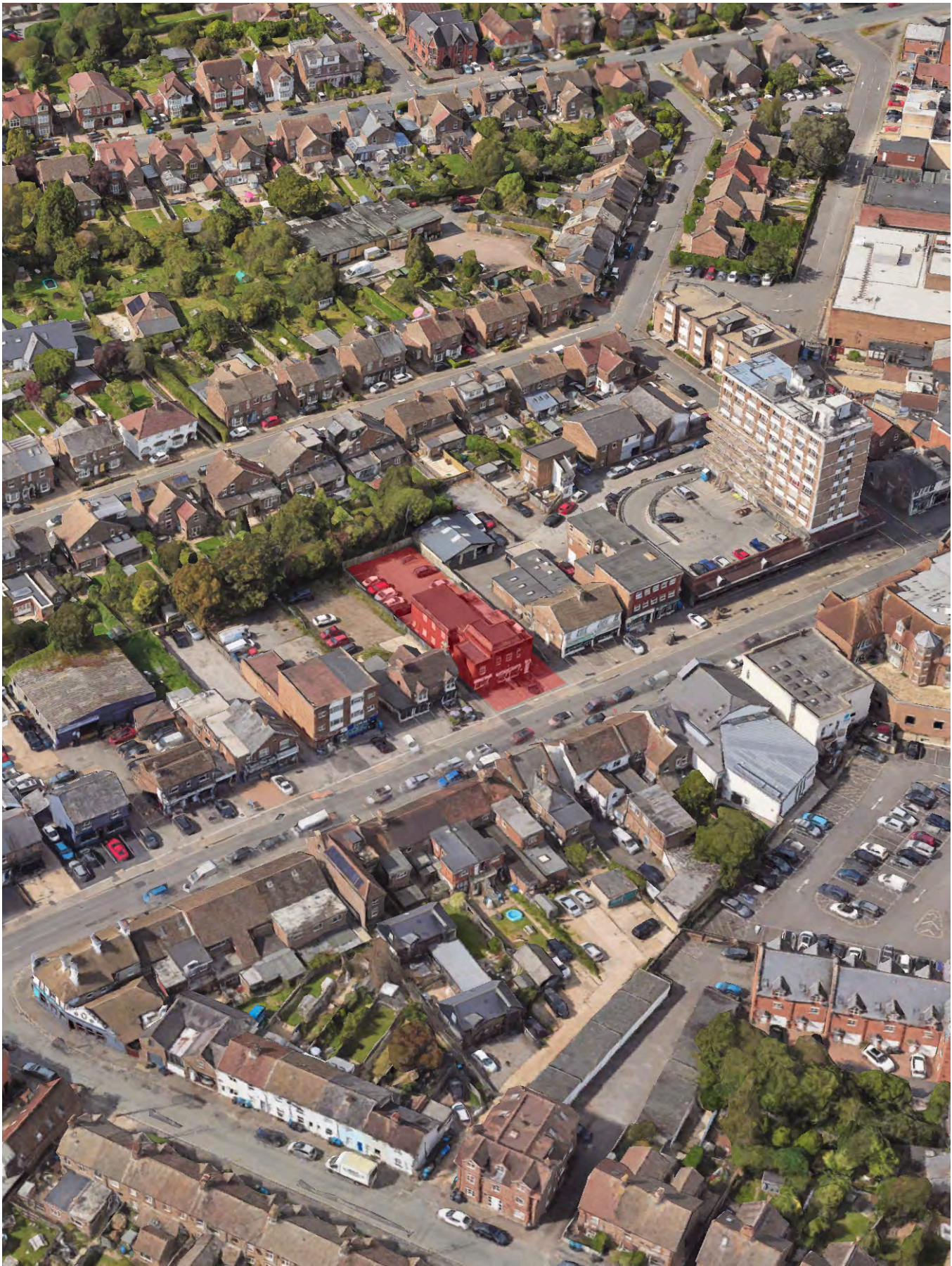
Google Earth perspective view looking northeast across Sussex Road, with site highlighted in red
