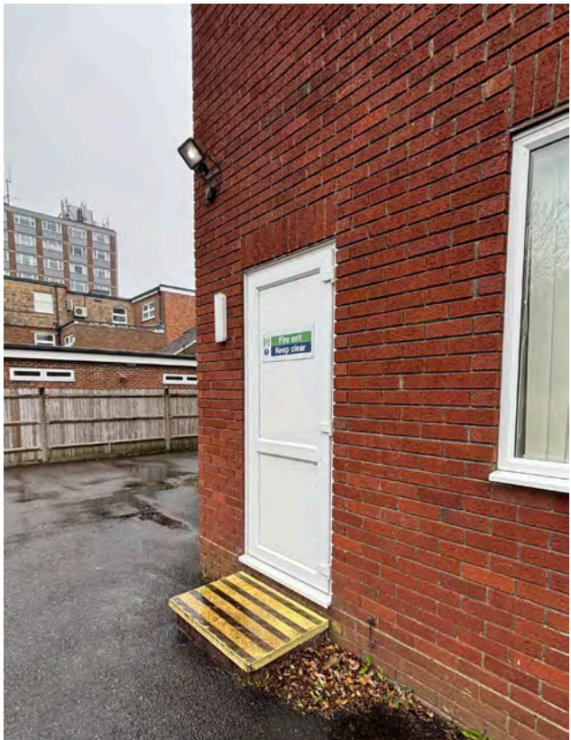
External door opening onto existing car park to the rear
