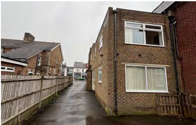
Extension to the north made in brown brick
