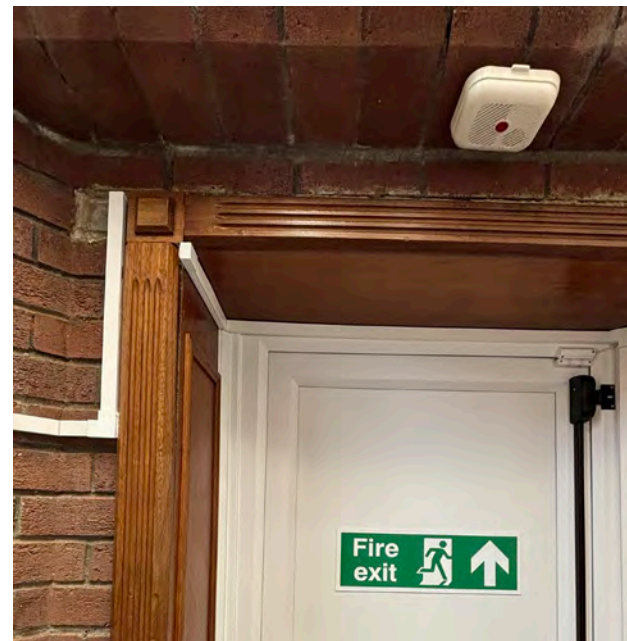
Decorative solid door reveal and architrave to entrance door in the stairwell
