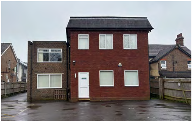
Rear elevation showing roof with sloped edges and what appears to be fibre-cement tiling with the appearance of slate
