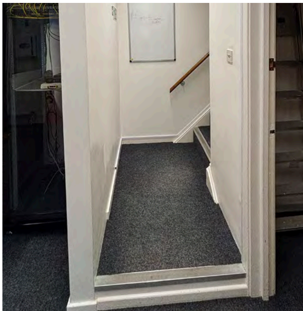
Large landing at Stair 2
