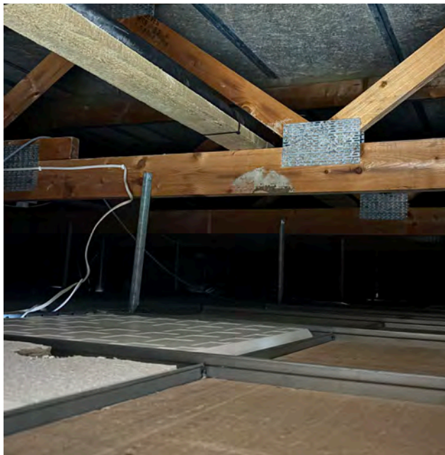
Suspended ceiling in conference room on first floor
