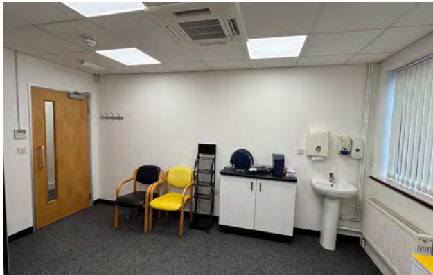
A typical cellular office at ground floor
