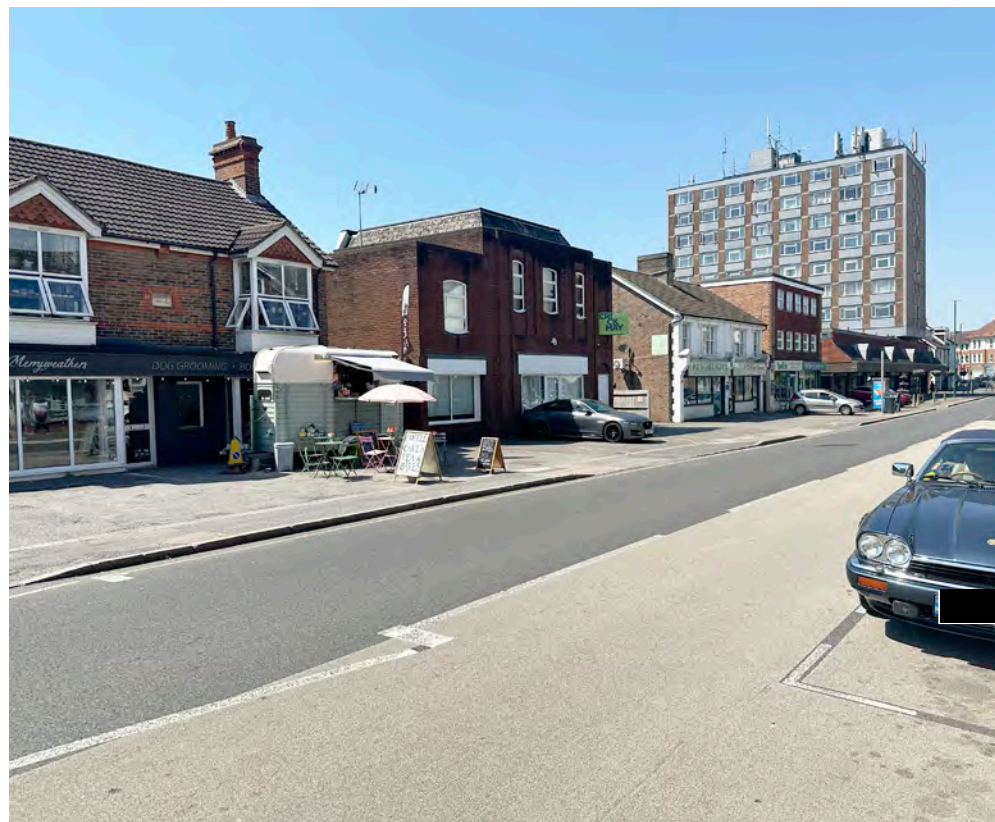
Site photo looking northwest across Sussex Road towards the existing building
