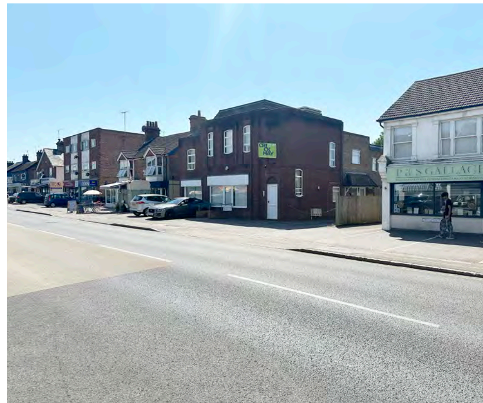
Site photo looking southwest across Sussex Road towards the existing building
