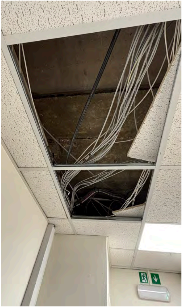
Typical suspended ceiling with services above, ground floor
