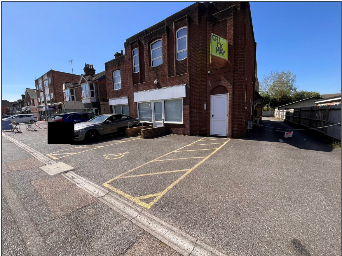
Photograph 1 Site Frontage at Sussex Road as Existing
