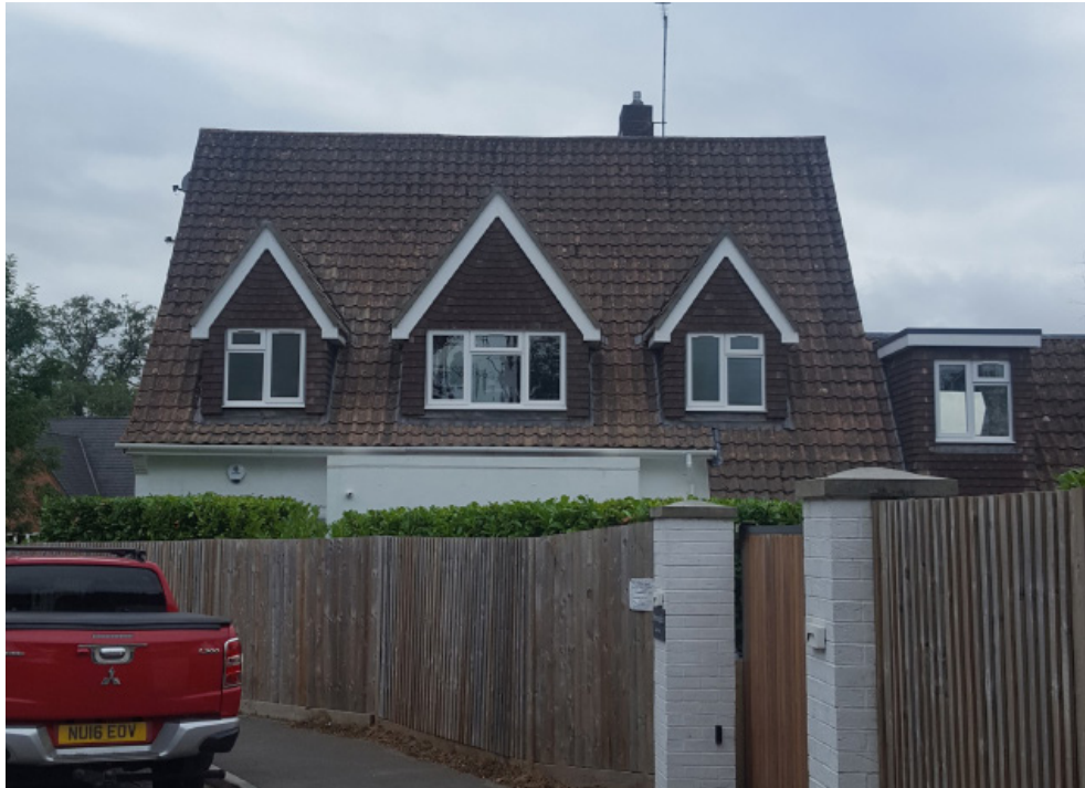
Approval in Keymer Road under construction
