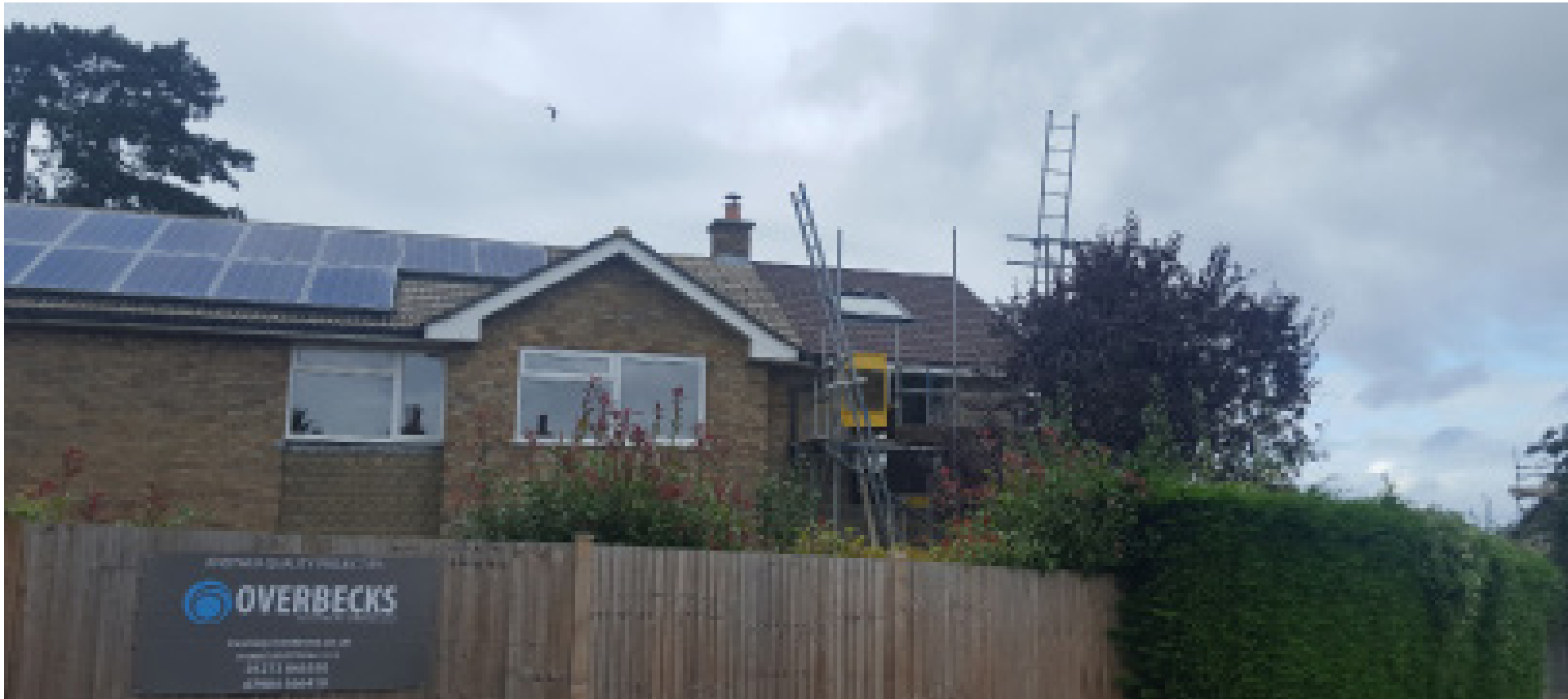
Approval in Birchwood Grove under construction
