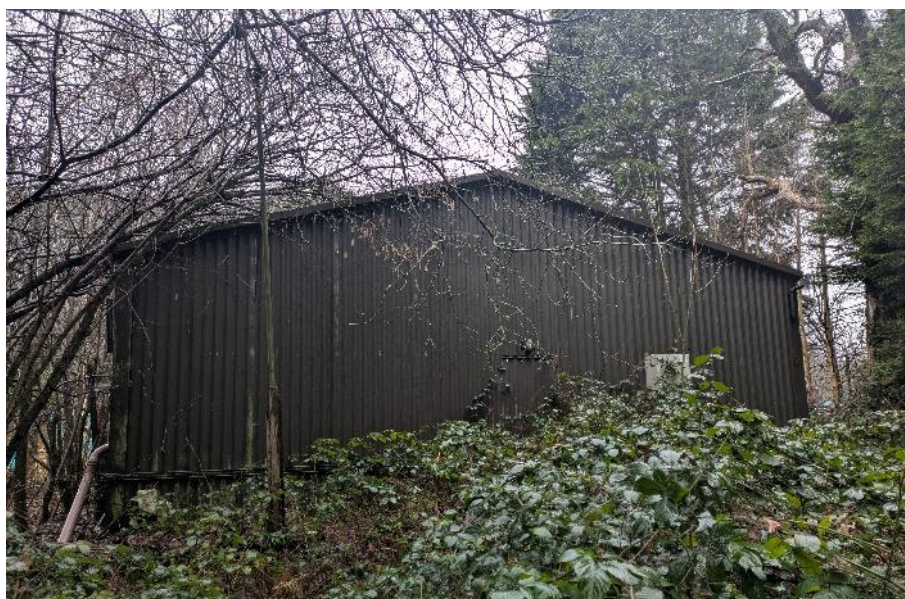
Plate 3: A photograph of the south-eastern elevation of the building B1 .
