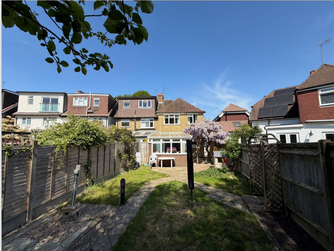
Rear elevation of 50 Stanford Avenue
