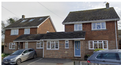
Photos above show existing houses in Horsted Keynes with brick finish at ground floor and clay tile hanging at first floor.
