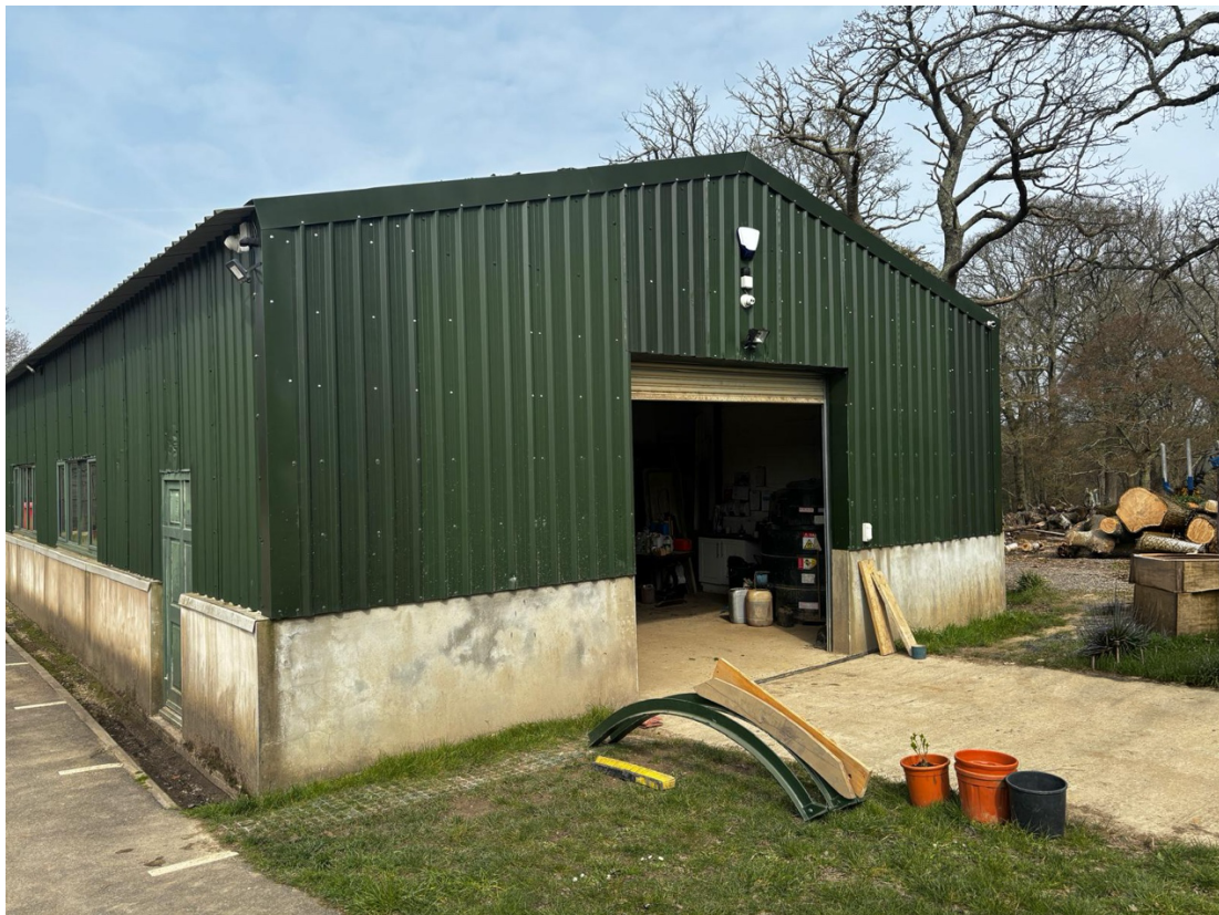
View of Existing Shed at Greentree Farm
