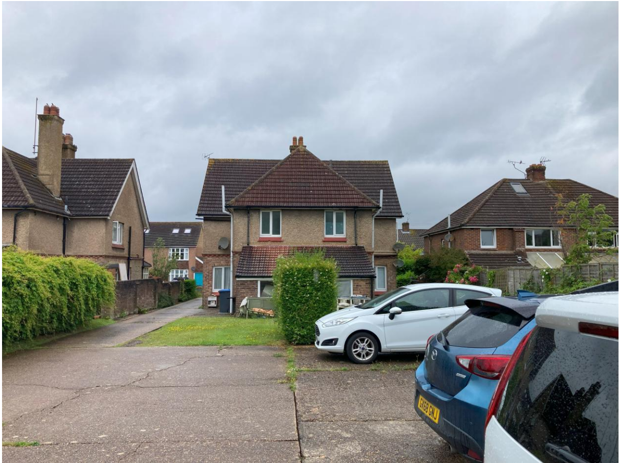
Image 03 – Rear elevation of no. 12 & 14 viewed from rear of site
