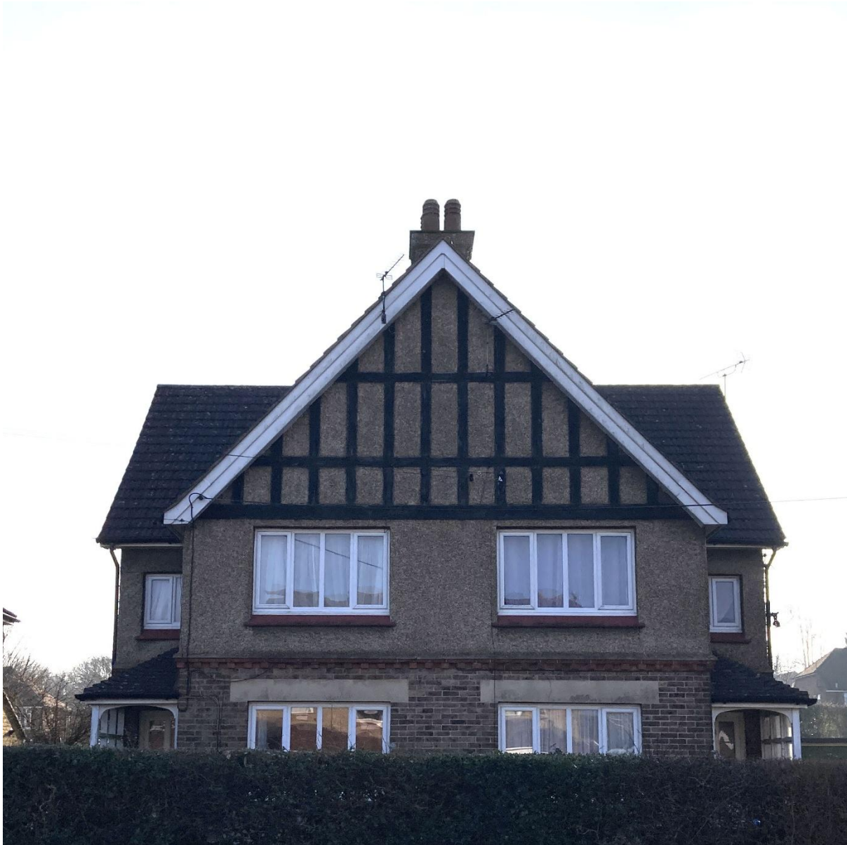
Image 07 – No. 14 and no. 12 front elevation viewed from Eastern Road
