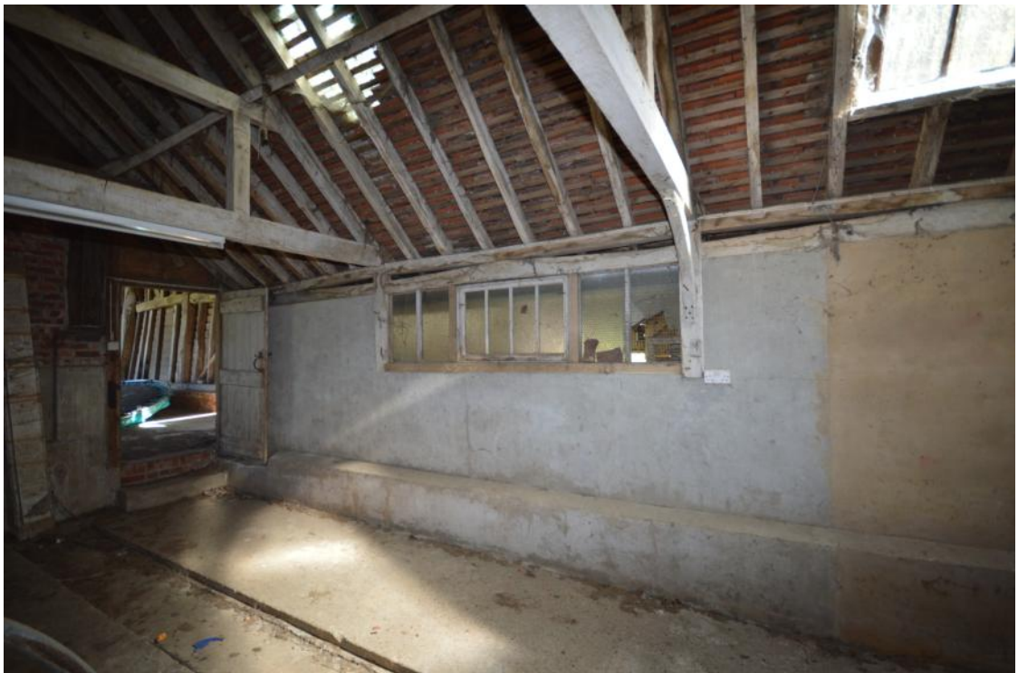
Plate 36: The east front of building B2a showing the truncated posts, head-braces, bressumers and head-plates
