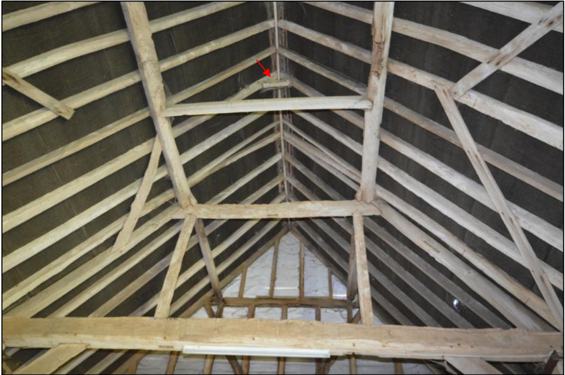
Plate 24: The north end of the barn showing the high-set collar (arrow) that had supported the half-hipped roof terminal at that end of the building prior to the addition of bay 5 in the 17 th century
