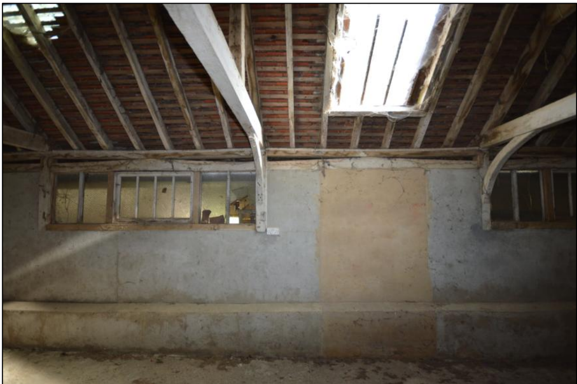
Plate 33: The west side of B2a showing the former open front evidence: the head-plate below the bressumer/flying plate, the posts between the bays, and the nailed-on head-braces
