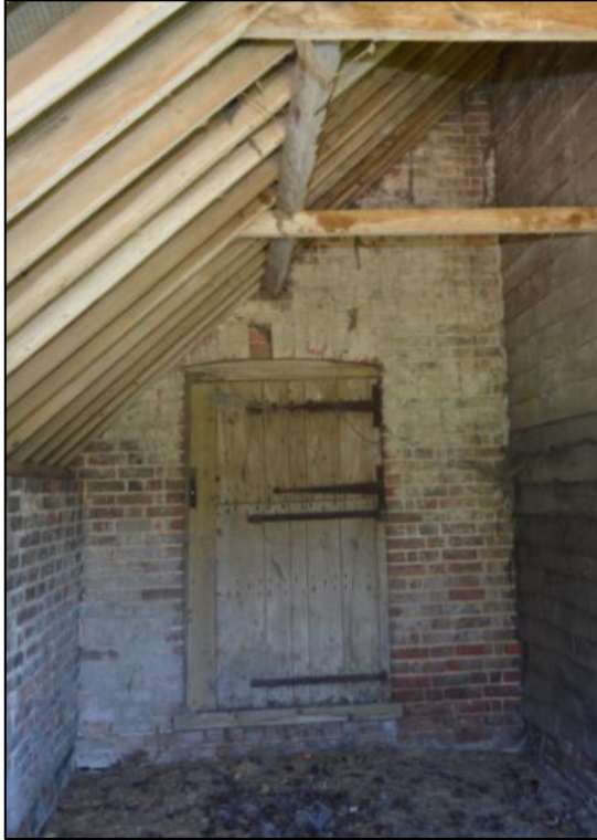
Plate 15: The doorway in the east elevation of the north outshot (B3)
