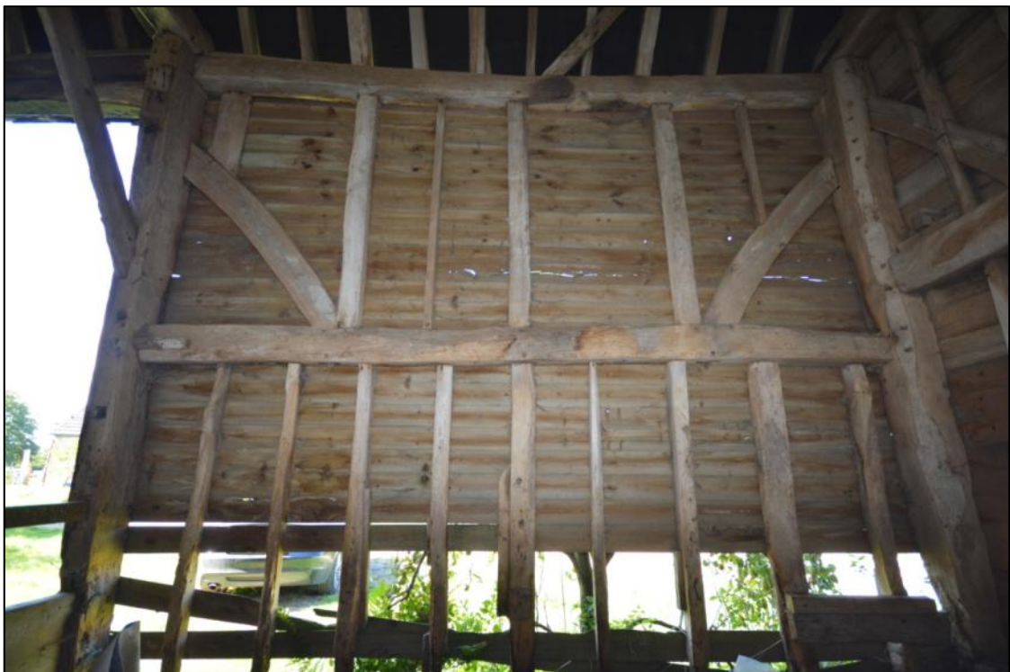
Plate 20: The wall construction of the west elevation (bay 1), without intermediate full-height posts
