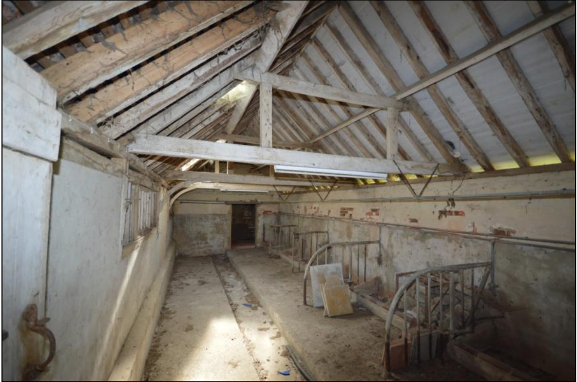
Plate 35: Roof structure and typical roof truss
