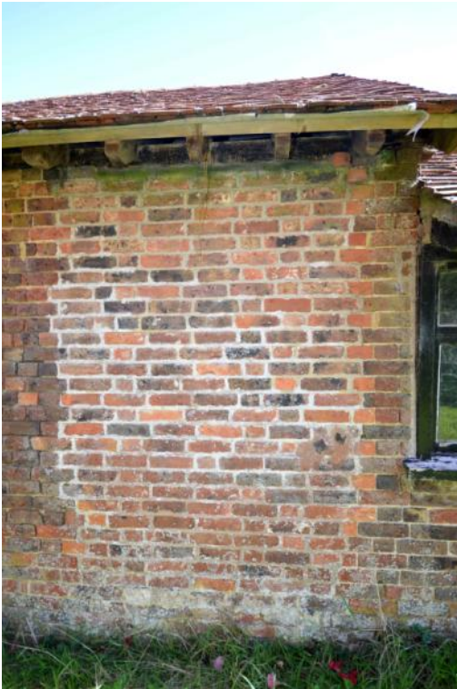
Plate 31: The evidence of a blocked doorway in the west elevation of bay 4 (B2a)
