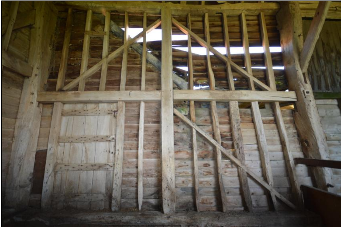
Plate 28: The much rebuilt eastern elevation of bay 1 (the door is a later insertion removing two of the 19 th century studs to accommodate it)
