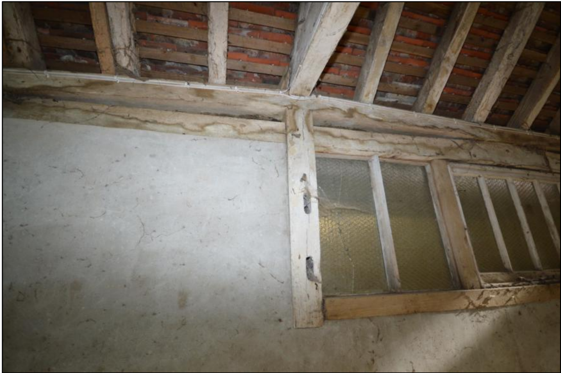
Plate 30: Detail of the mortises on the post between bays 1 and 2 of B2a, indicative of a partition
