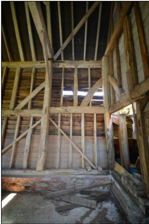
Plate 26: The east elevation of bay 4, added to the south end of the barn during the 17 th century
