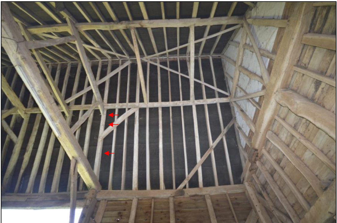
Plate 25: The west slope of the roof over bay 1 showing the lash marks on the principal rafter of the T2 truss, left from the original thatched roof cover (indicated by arrow)
