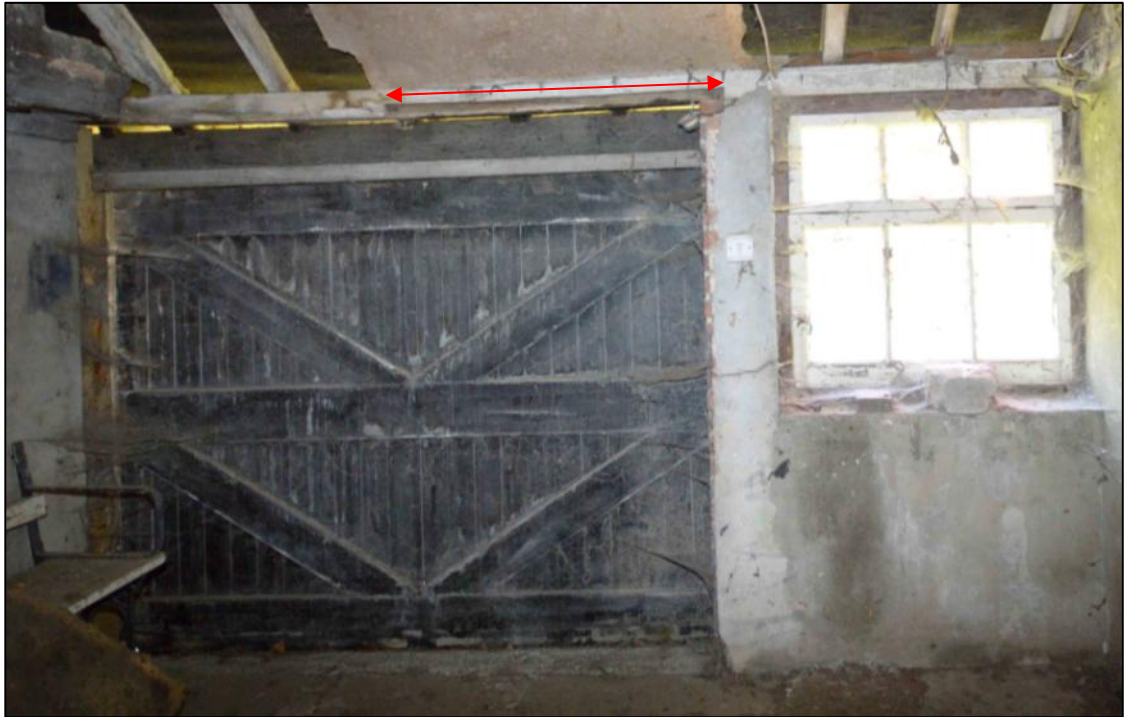
Plate 34: Bay 5 (B2b) showing evidence of the widening of the doorway (arrow)
