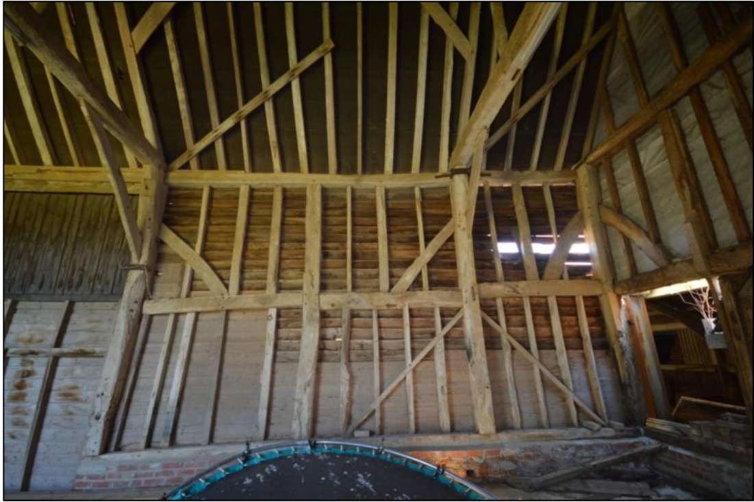
Plate 21: The east elevation, south end showing the wall construction with intermediate full-height post (bay 4)
