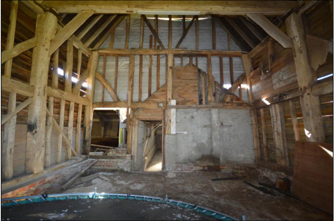
Plate 27: The much altered south end of the barn, retaining the interrupted girt, upper central studs, foot-braces and central full height stud of the original 17 th century extension
