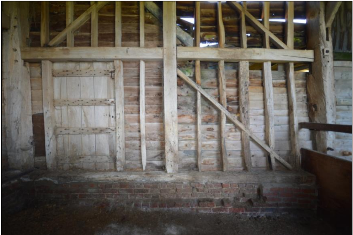
Plate 12: The doorway inserted into the rebuilt eastern elevation of bay 1 after the 19 th century rebuild
