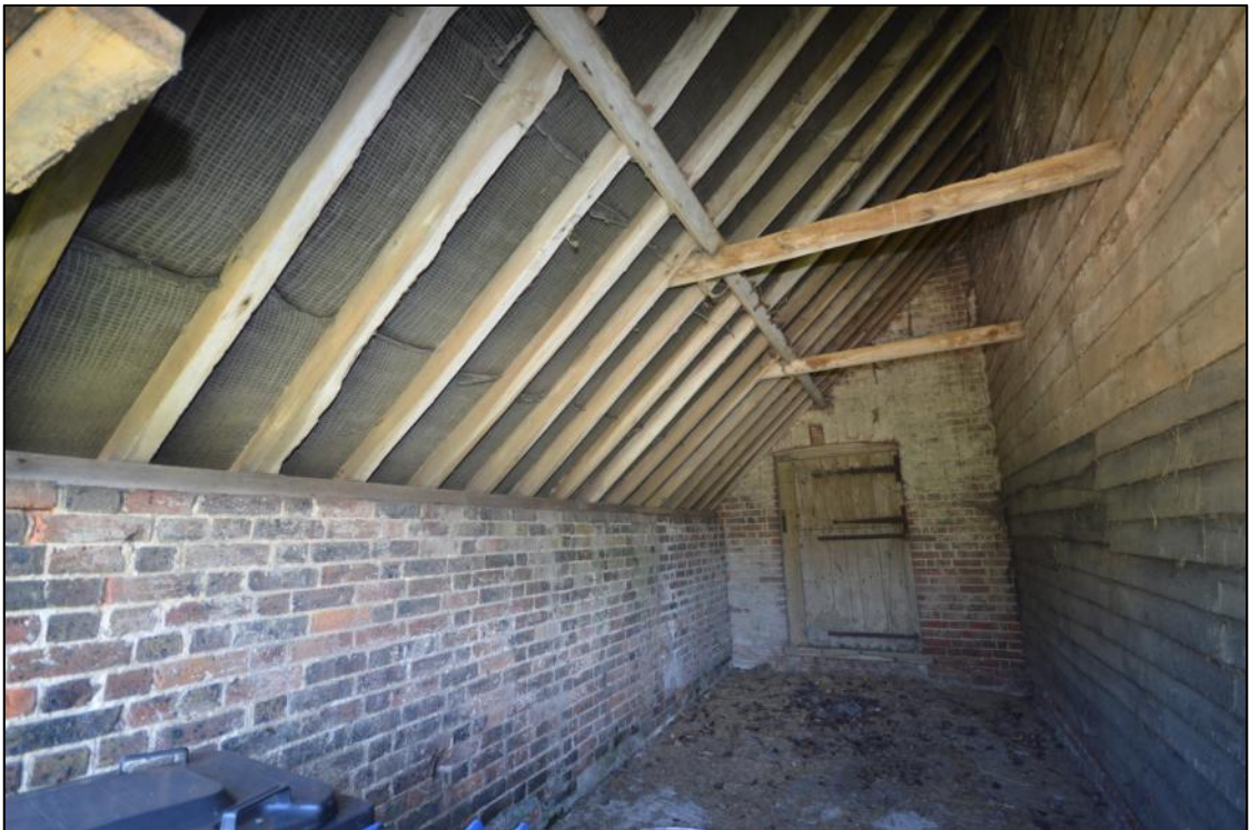
Plate 38: The interior of B3 as it abuts the barn, looking towards the inserted brick partition with its integral doorway
