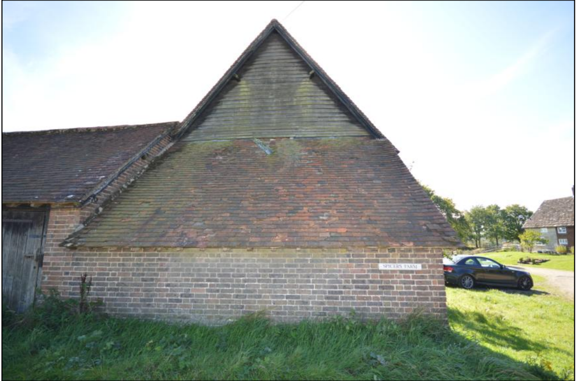
Plate 37: The north end of the barn and building B3
