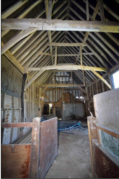
Plate 23: View towards the south end of the barn showing the open trusses flanking the wagon entrance
