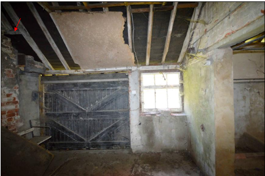
Plate 32: The interior of bay 5 (B2b) showing the scars for a flue and the jointed-in trimmer in the rafters (arrow)
