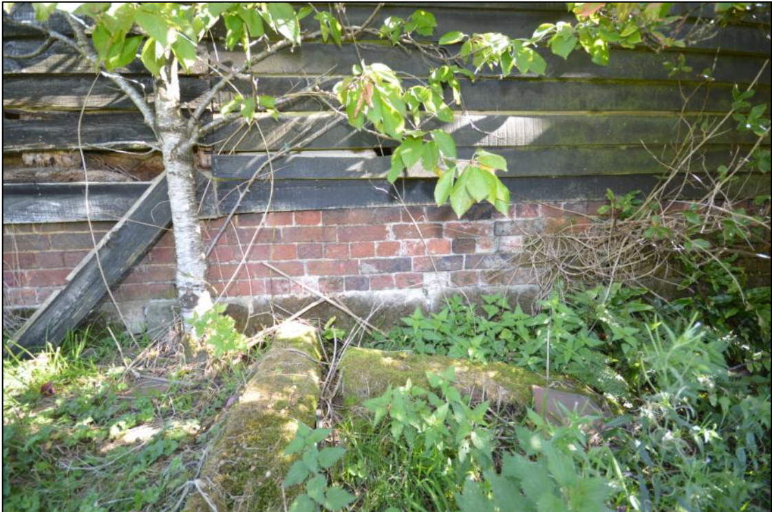
Plate 29: Detail of the brick plinth surmounting the masonry base on the western side of the barn (bays 3 and 4)
