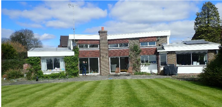
Fig. 1 – Rear (south side) of existing house, viewed from lawn
