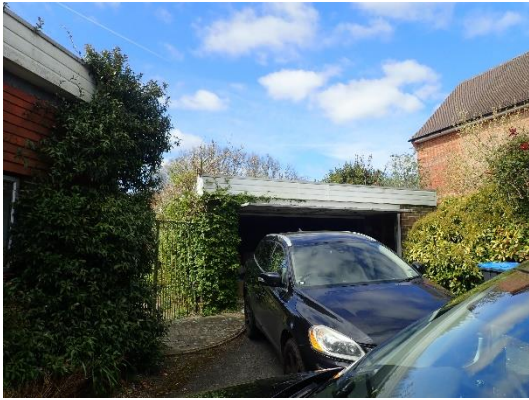
Fig. 9 – Garage to NW of house
