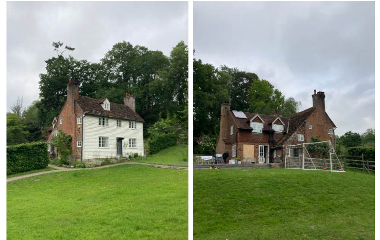
East and south elevations (left) and north and 1986 extension (right) of Burstow Cottage.
