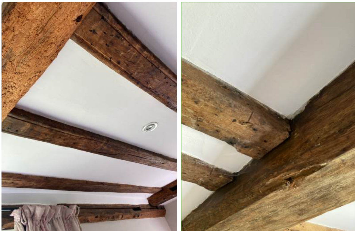
Late C17 beaded joists (left) and C16 joists with curve-stepped chamfer stops (right).
