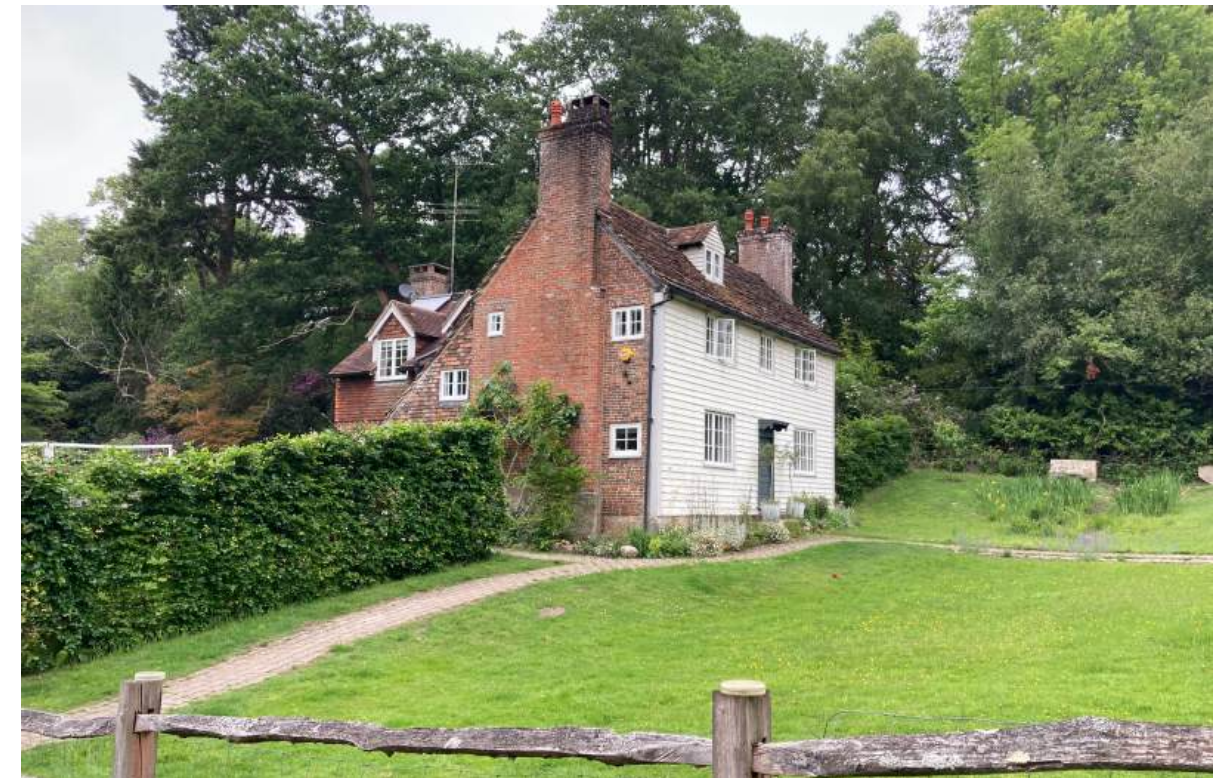
View of Burstow Cottage from its private driveway. Note the modern stack is partially visible.
