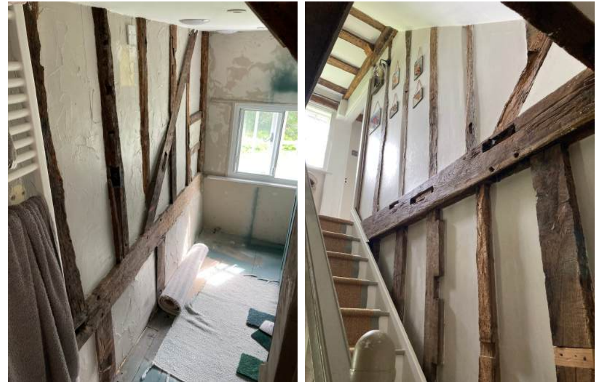
Examples of exposed framing throughout the house. Note the presence of empty mortices which indicate reclaimed timber.
