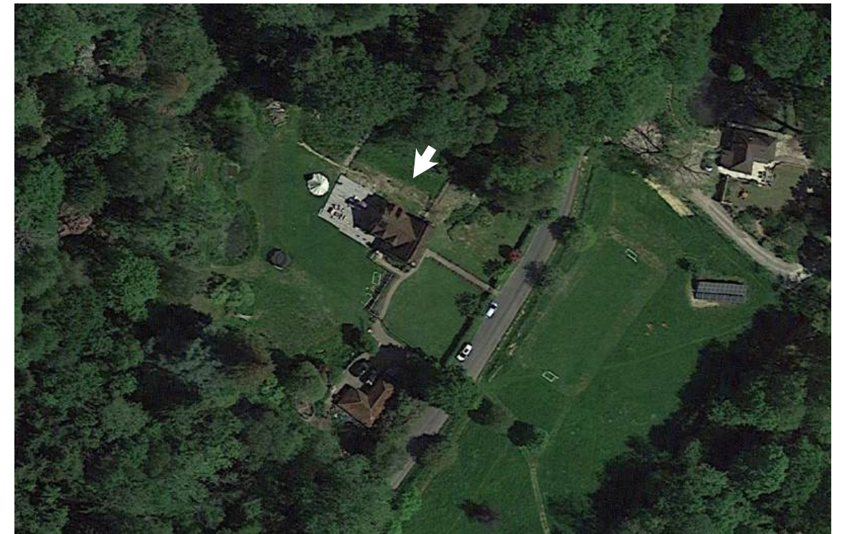
Satellite View of Burstow Cottage, 2021 (© Google Earth).
