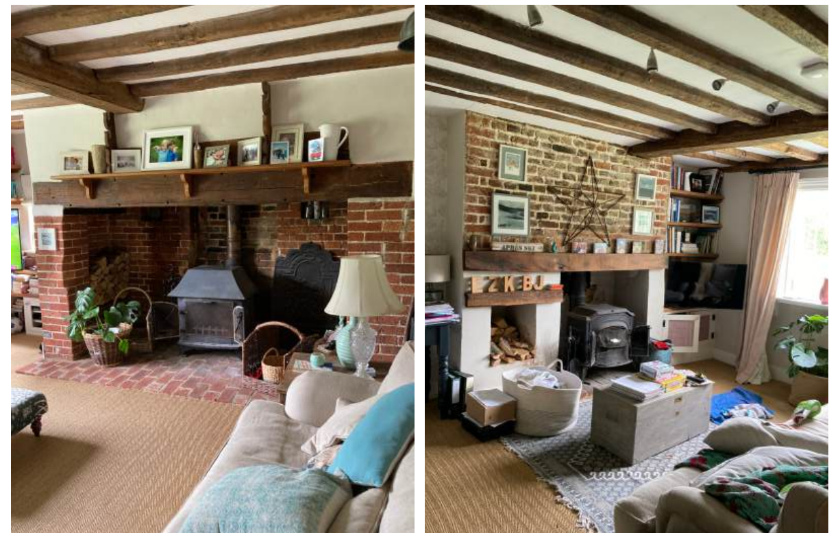
Inglenook serving the former kitchen (left) and altered fireplace serving the former parlour (right).
