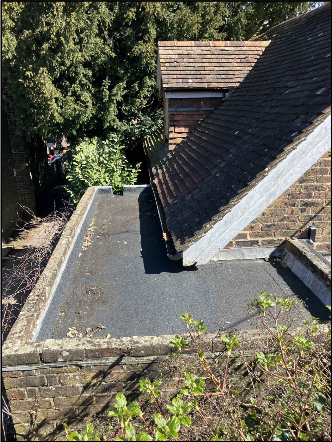
Reference Image: Existing felt roof
