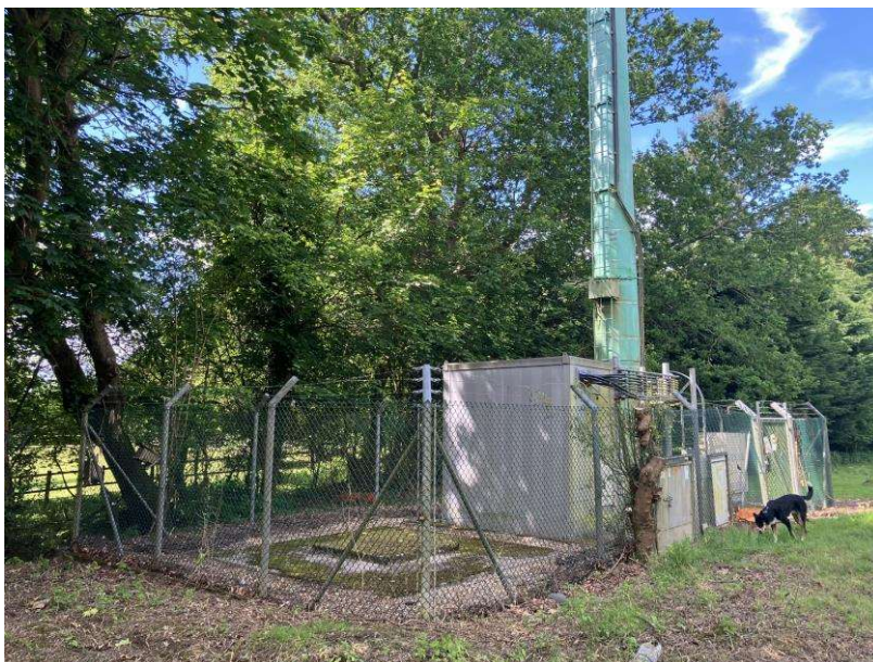
Photo of existing telephone mast and infrastructure and concrete base.
