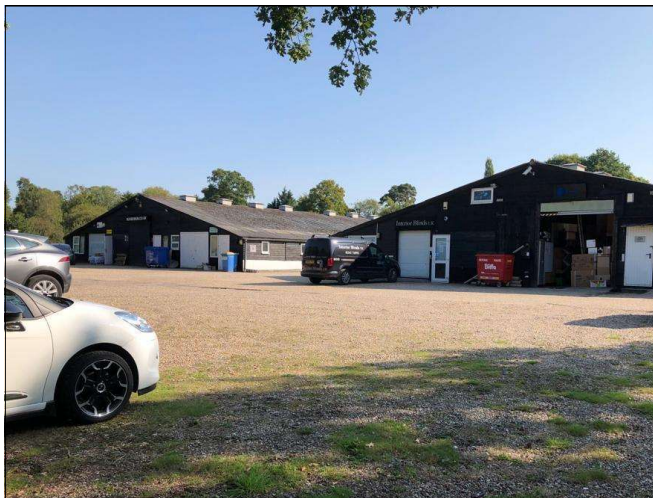
Example of wood-clad small business workshops at Barns Court and ancillary gravelled parking
