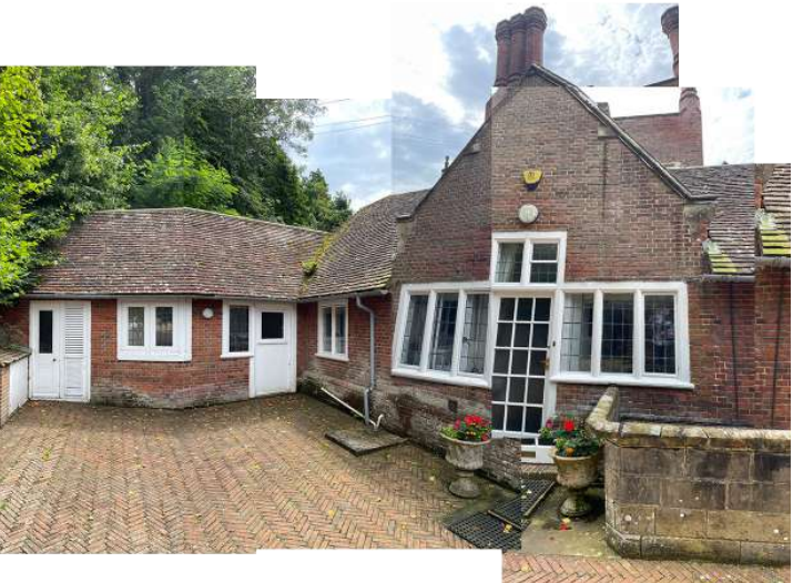
A1 - External view of services courtyard
