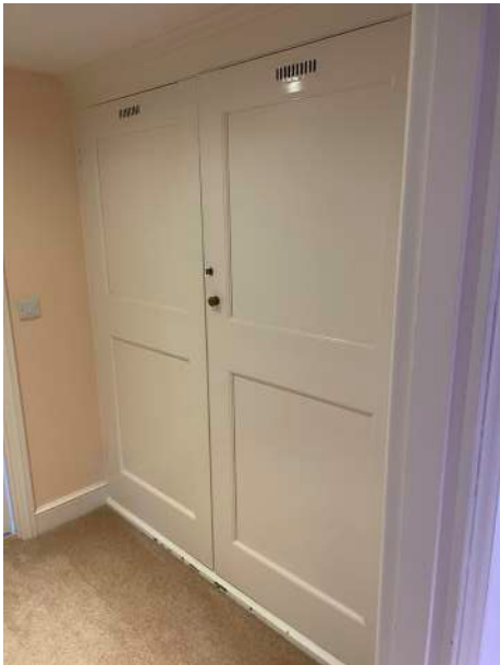
K Wall (right) to be removed
