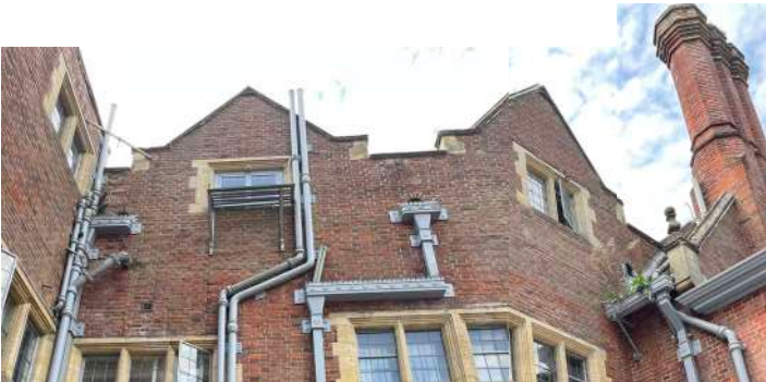
C2 - View of existing elevation from courtyard
