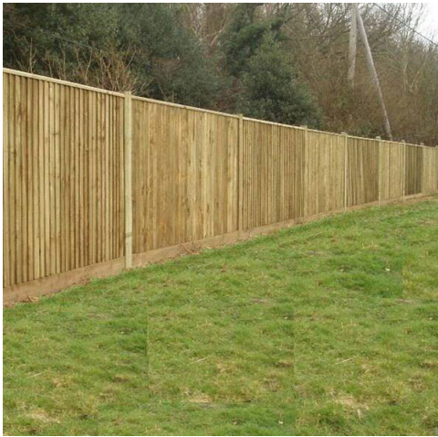
Closeboarded timber fence
