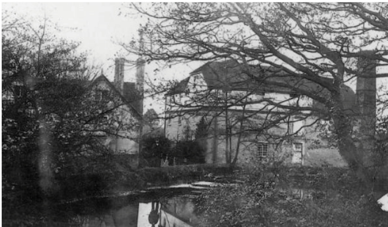
rear of Mill House (listed in 1983)
