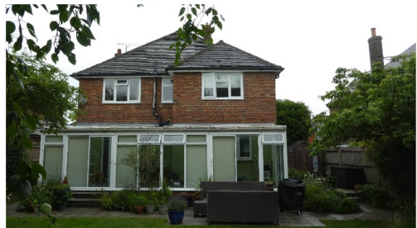
Figure 2 - Rear of property
