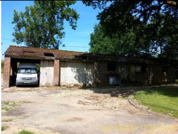
Figure 14: B3b – east elevation. The roof is single skinned and of corrugated asbestos construction. The building is open due to large doors and missing roof panels.
