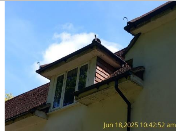
Figure 13: B2 – dormer window close-up. Only one dormer window on B2 is clad in hanging tiles.
