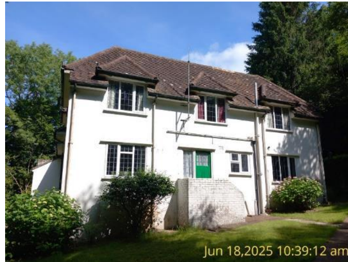
Figure 2: B2 (the Lodge) – south elevation.
