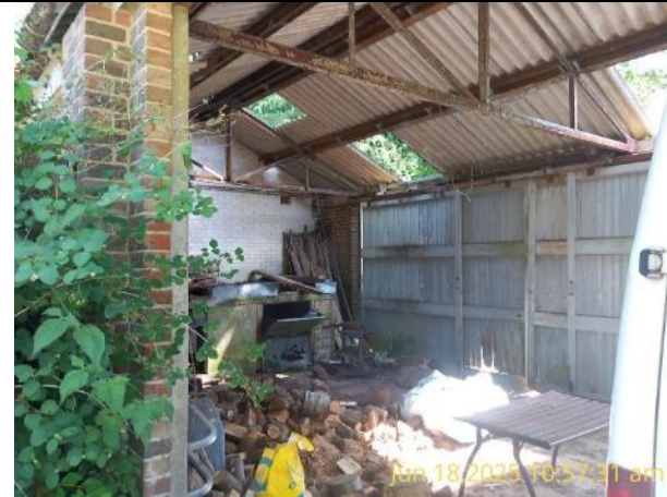
Figure 23: Interior of B3b.
