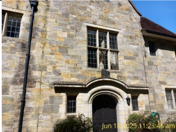
Figure 4: B1 – east elevation. Doors and window frames are of timber construction and are tight-fitting to the brickwork.
