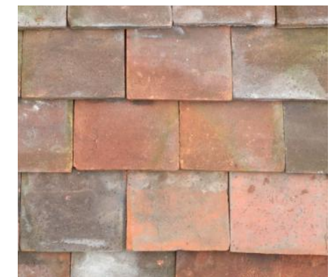
Reclaimed plain red clay roof tiles to match existing.
