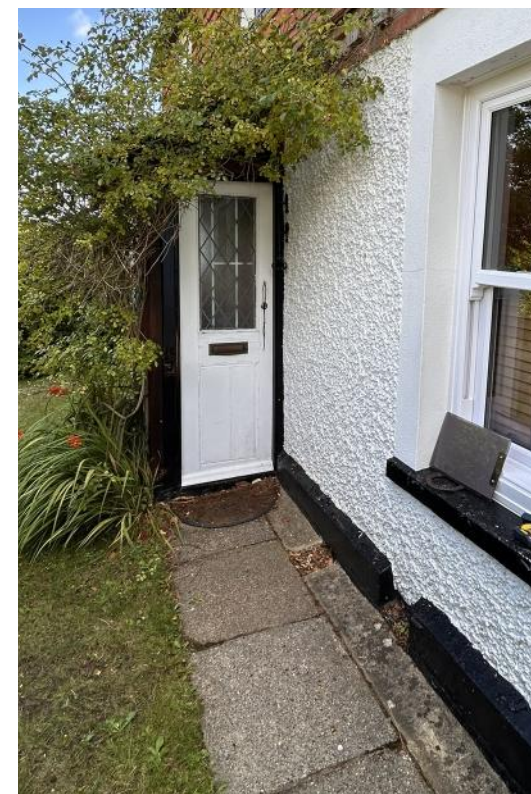
View of the South entrance end of the porch from within the front garden.
