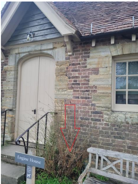
Photo 3: Approximate location of insertion point for water pipe (red arrow).
