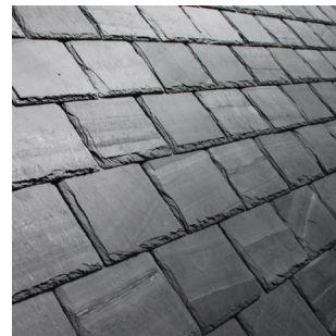
Natural Welsh Roofing Slate
