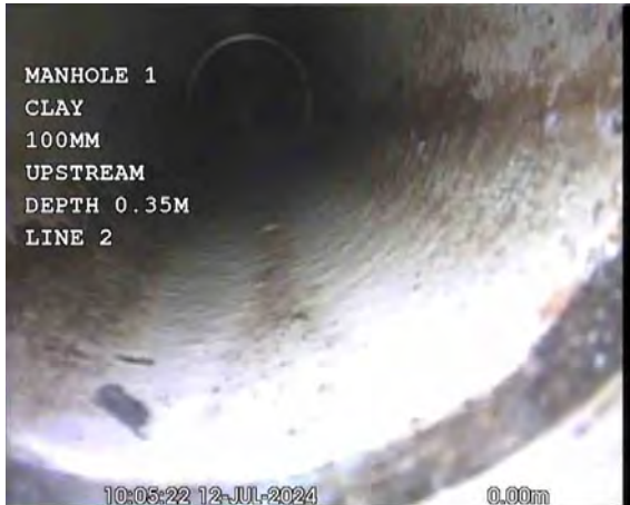
W_CX_195b9a80-0444-4a50-909c-826c72029cfe_20240725_090339_479.jpg, 00:00:20, 0.00 m Start node, manhole, reference: MANHOLE 1 (MH1)
