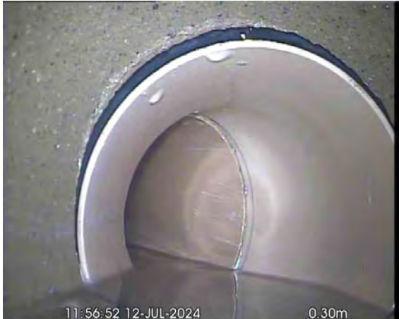
MH2X_b91b3937-c37a-452d-9c54-7c35945f681d_20240725_092617_600.jpg, 00:00:56, 0.30 m Material changes to polyvinyl chloride
