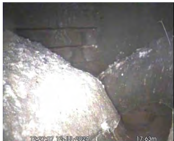
MH5X_14be63c4-1844-4b3b-8d9d-02ec269f888d_20240725_095012_235.jpg, 00:02:35, 17.63 m Finish node, manhole, reference: MANHOLE A (MHA), (DAWN RISE ROAD)
