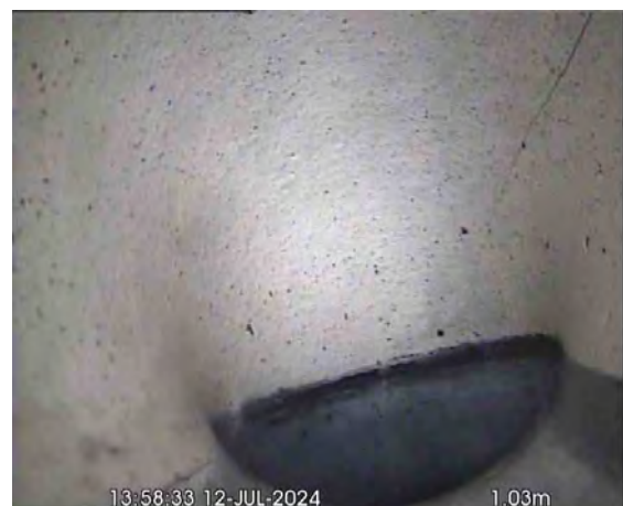
GULLYX_c67647b2-92e2-40c2-a9d7-fb213594d517_20240725_100025_314.jpg, 00:00:28, 1.03 m Finish node, gully, reference: GULLY
