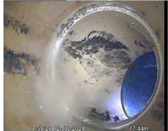
MH2X_ecbc01d4-5401-430c-a4cc-4e8128ef4209_20240725_093238_853.jpg, 00:02:20, 17.44 m Line deviates right
