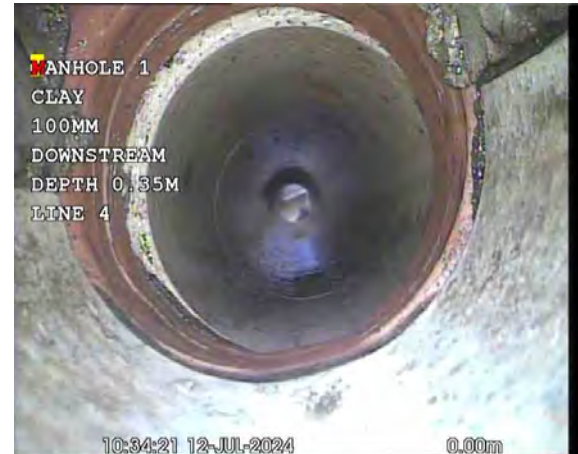
MH1X_e19867f0-c5b3-4e72-bae8-ed380d85fbba_20240725_090929_878.jpg, 00:00:20, 0.00 m Water level, 0% of the vertical dimension
