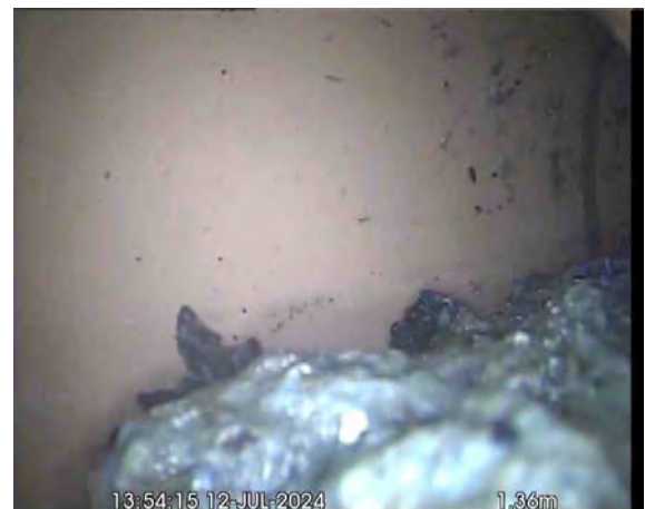
SVPX_7b6e8666-8fb9-44b5-8e1a-aafe5937a5df_20240725_095424_962.jpg, 00:01:07, 1.36 m Line deviates right
