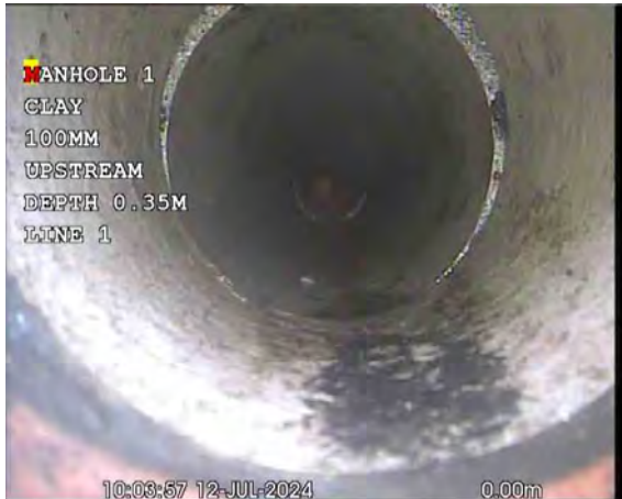
GULLYX_73fdf716-c185-4359-baea-e2cfaeeb6cce_20240725_090127_925.jpg, 00:00:34, 0.00 m Start node, manhole, reference: MANHOLE 1 (MH1)
