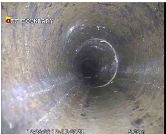
MH5X_7a719423-7b10-4cb5-9e10-35a6d7d11f95_20240725_094749_245.jpg, 00:01:36, 5.06 m General remark, **BOUNDARY POINT**
