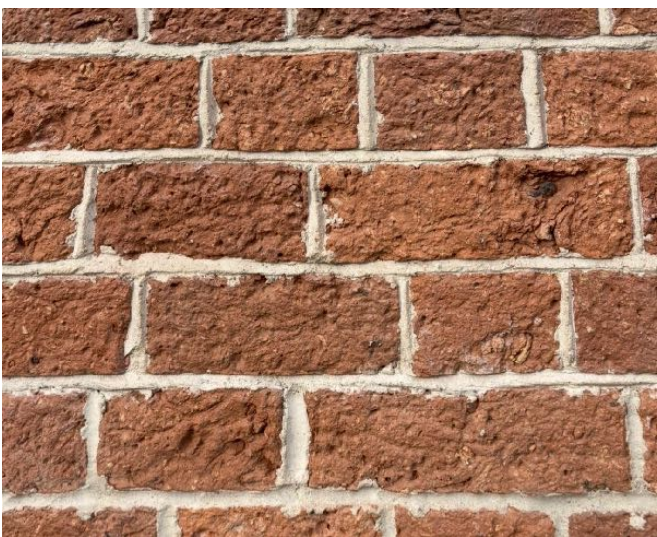
ON SITE LIME MORTAR TEST PANEL - BUCKET HANDLE POINTING PROPOSED
