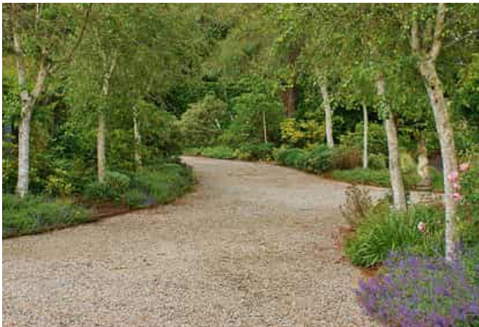
■ Hoggin, 80-100mm self binding clay-gravel base with a 50mm gravel wearing course. Location: Lake and woodland area
