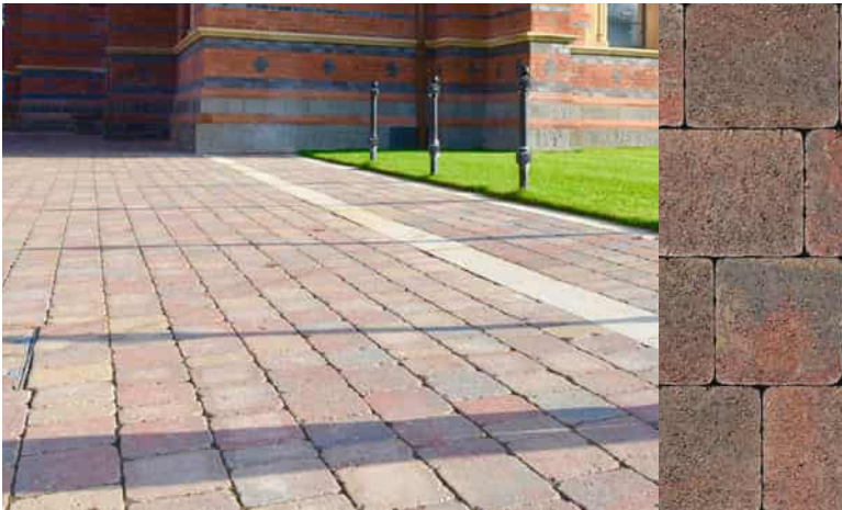
■ Tegula concrete block paving in a three-size mix, 80mm thickness. Colour: Heather. Laid: Stretcher bond. Location: Shared surface - in front of CFB
