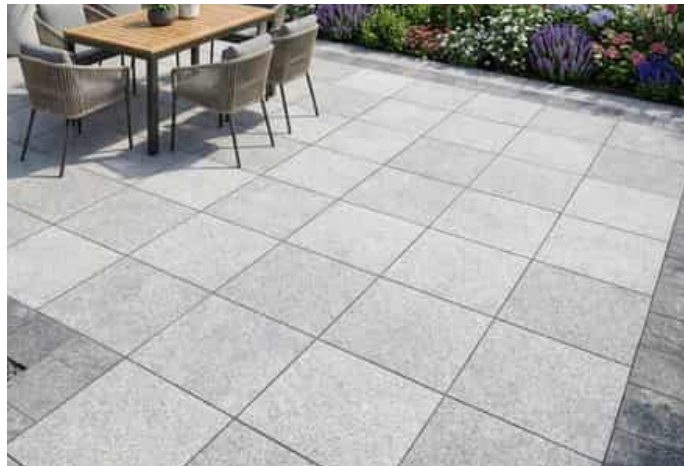
■ Flag concrete paving, natural granite aggregate. 400x400x50mm. Colour: Silver grey. Laid in stack bond. Location: Private amenity/ rear garden
