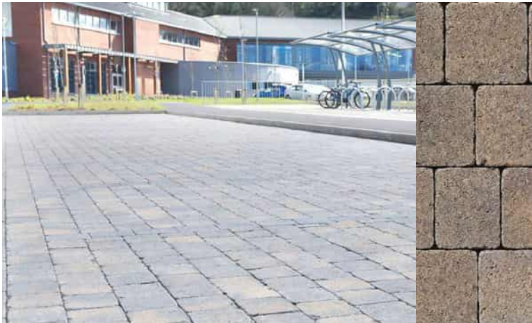
■ Tegula concrete block paving in a three-size mix, 80mm thickness. Colour: Bracken. Laid: Stretcher bond. Location: Parking areas
