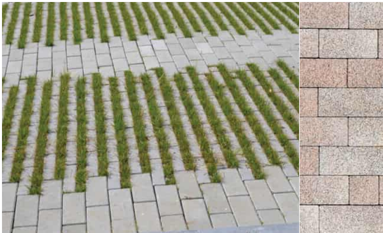
■ Linear green blocks, paving with 40% surface growing area, 100x300x100mm. Colour: Pink/ Light red Location: Refuse and emergency vehicle access and turning head
