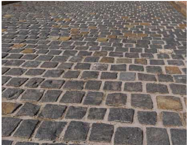
■ Granite setts, 100x100mm. Colour: Natural. Laid: Stack bond. Location: Ramp to raised table/ pedestrian crossing and paving bands
