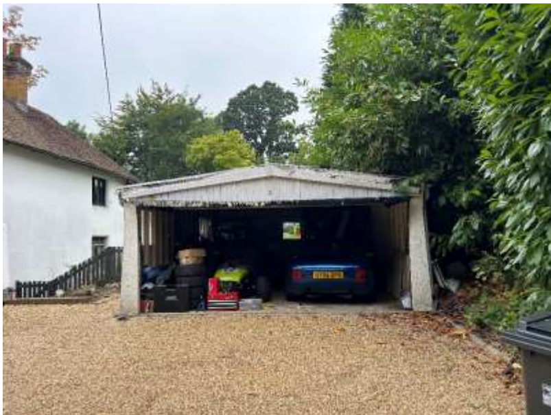
Photograph 2: The garage is of concrete construction with asbestos board pitched roof.
