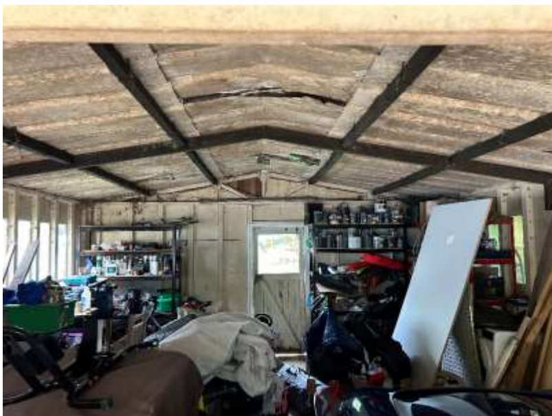
Photograph 3: Inside the garage. No evidence of bats was identified during the site walkover.
