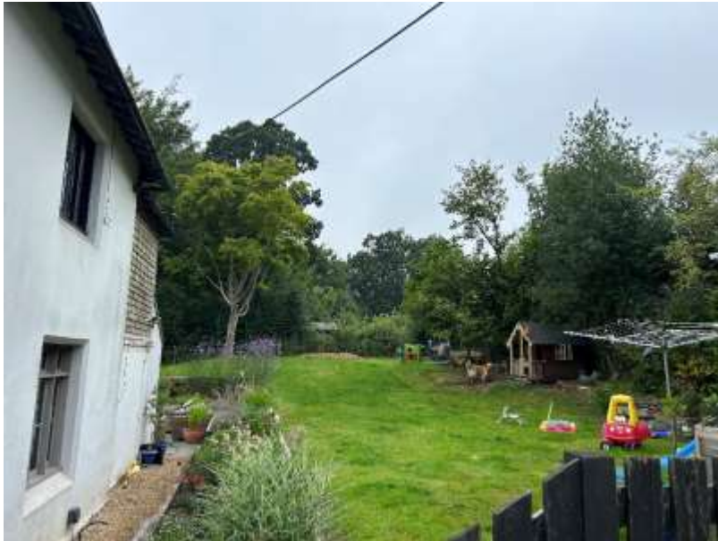
Photograph 1: The site comprises a residential dwelling with a detached garage and residential garden area to the rear.
