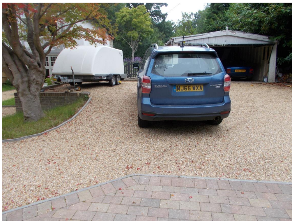
Photo 2: Permeable gravel access drive with double garage, workshop and store in the background.
