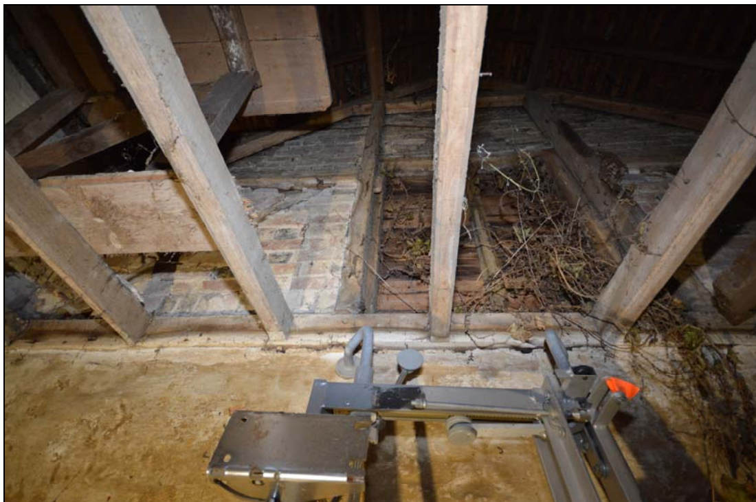
Plate 17: Detail of the T1 truss showing the lower tie-beam with joists, the junction of the northern of the two queen studs, and the junction of the stub-tie and the same queen stud, all jointed and pegged in place
