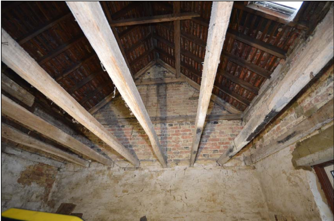
Plate 12: The interior of the building looking towards its eastern gabled end showing the wall fabric, finish, floor joists and roof construction
