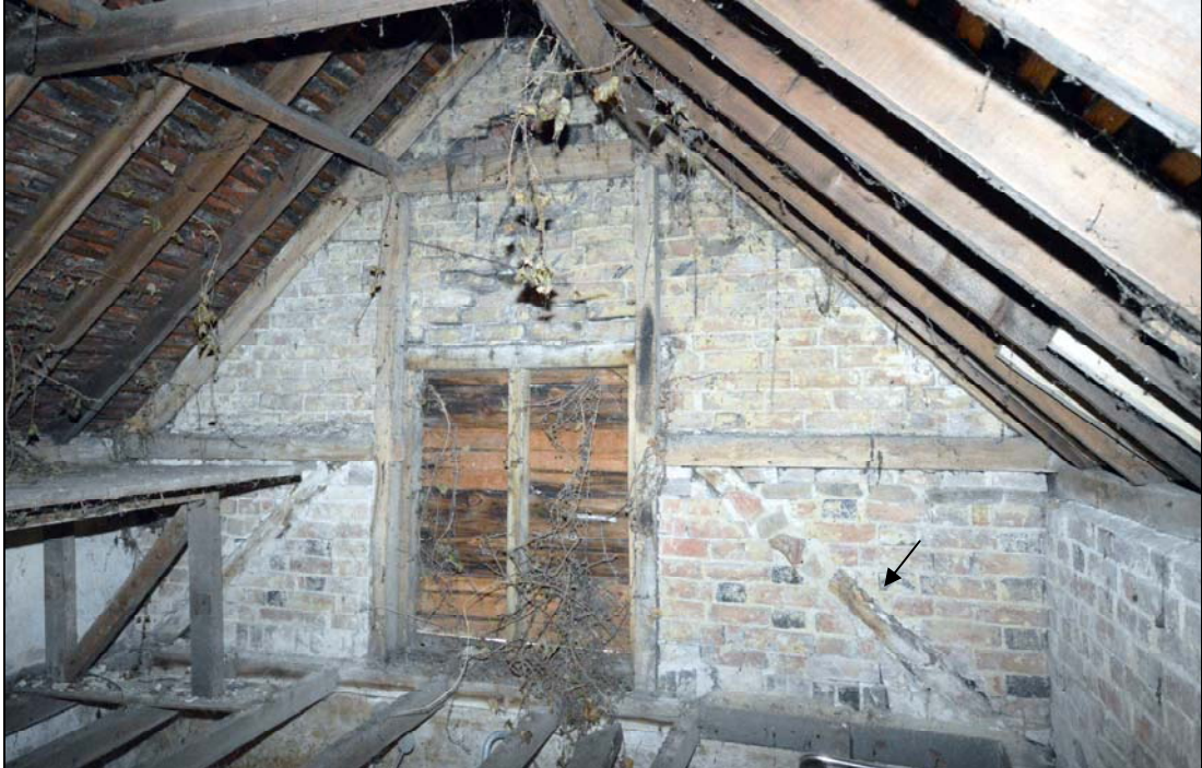
Plate 16: The T1 truss showing its well-carpented components and the infill where the southern of the two raking shores had been removed (arrow)
