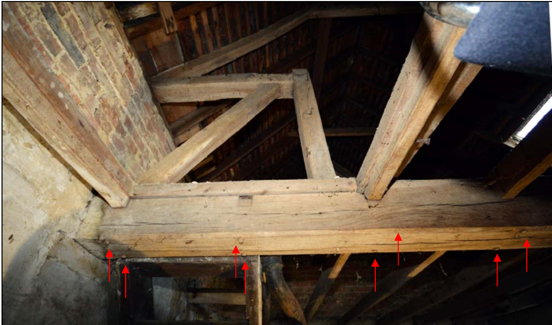
Plate 15: Detail of the north end of the cross-beam on its western side showing the joists or joist sockets (where removed) and the pegs that anchor them in place (arrows)
