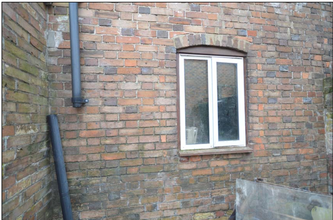
Plate 11: The Flemish bond brickwork of the walls of the ancillary range, note also the consistent coursing and lack of a straight-line joint at the junction with the north projection
