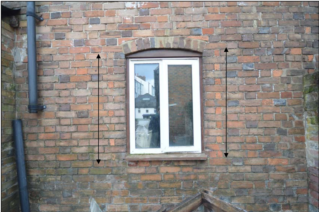
Plate 14: The integral window opening in the north elevation and the modern window inserted into it (queen closer columns indicated by arrow)
