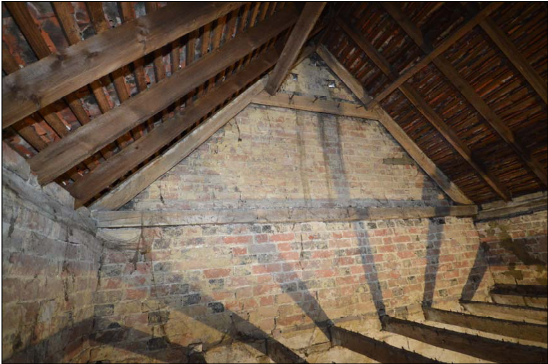
Plate 18: The western gable and the T3 truss
