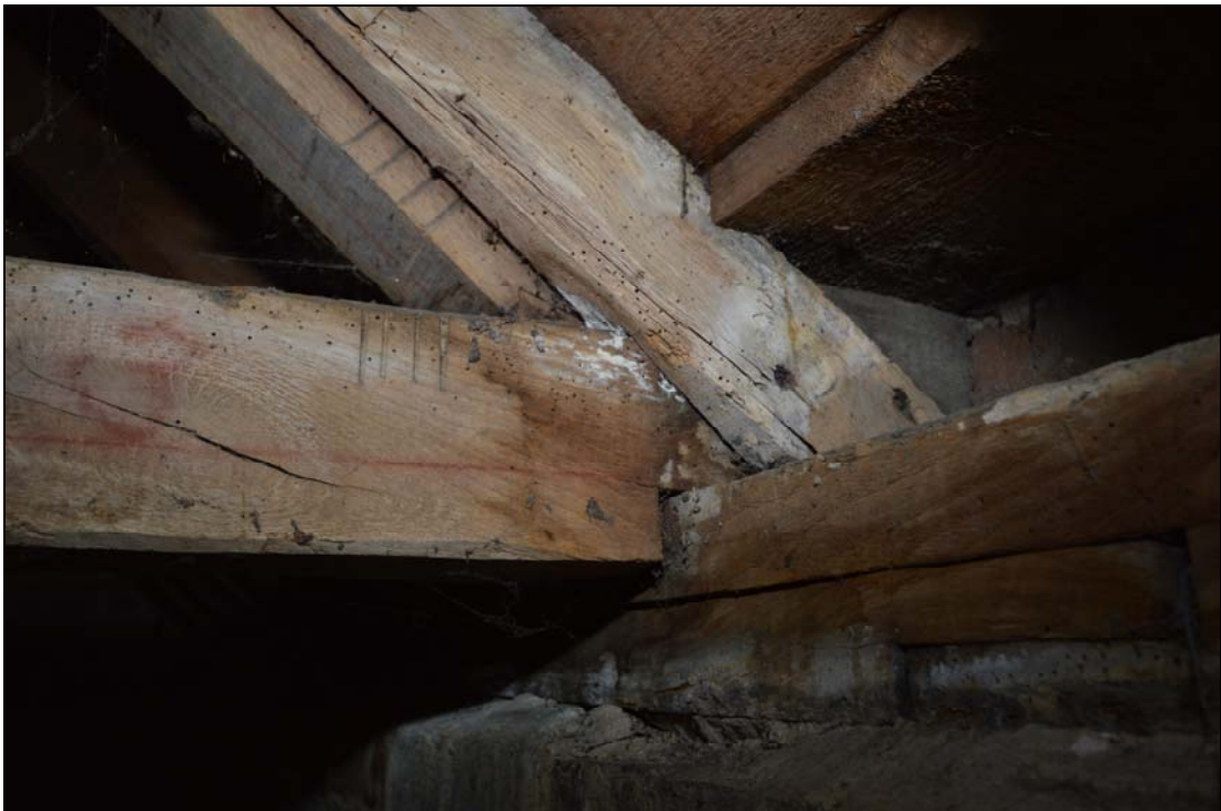
Plate 19: The junction of the principal rafter and the stub-tie at the south end of the T2 truss with the matching Roman numeral carpenter marks IIII
