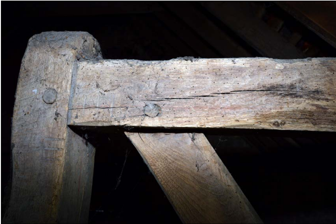
Plate 20: The junction of the posts and stub-ties of the T2 truss and the Roman numeral carpenter's marks III
