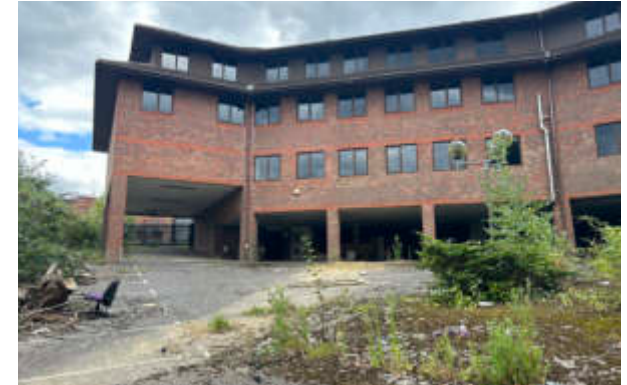
Existing parking at the rear of site
