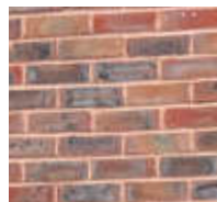
Red brick (existing and new infill).
