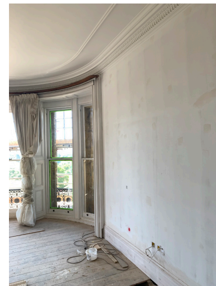
Example of cornicing and skirting retained
