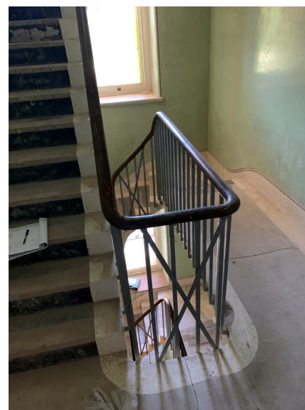
Example of existing stairwell balustrade retained
