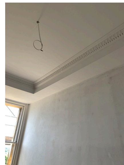
Dropped ceiling for ventilation (see comment on specific room occurrence)
