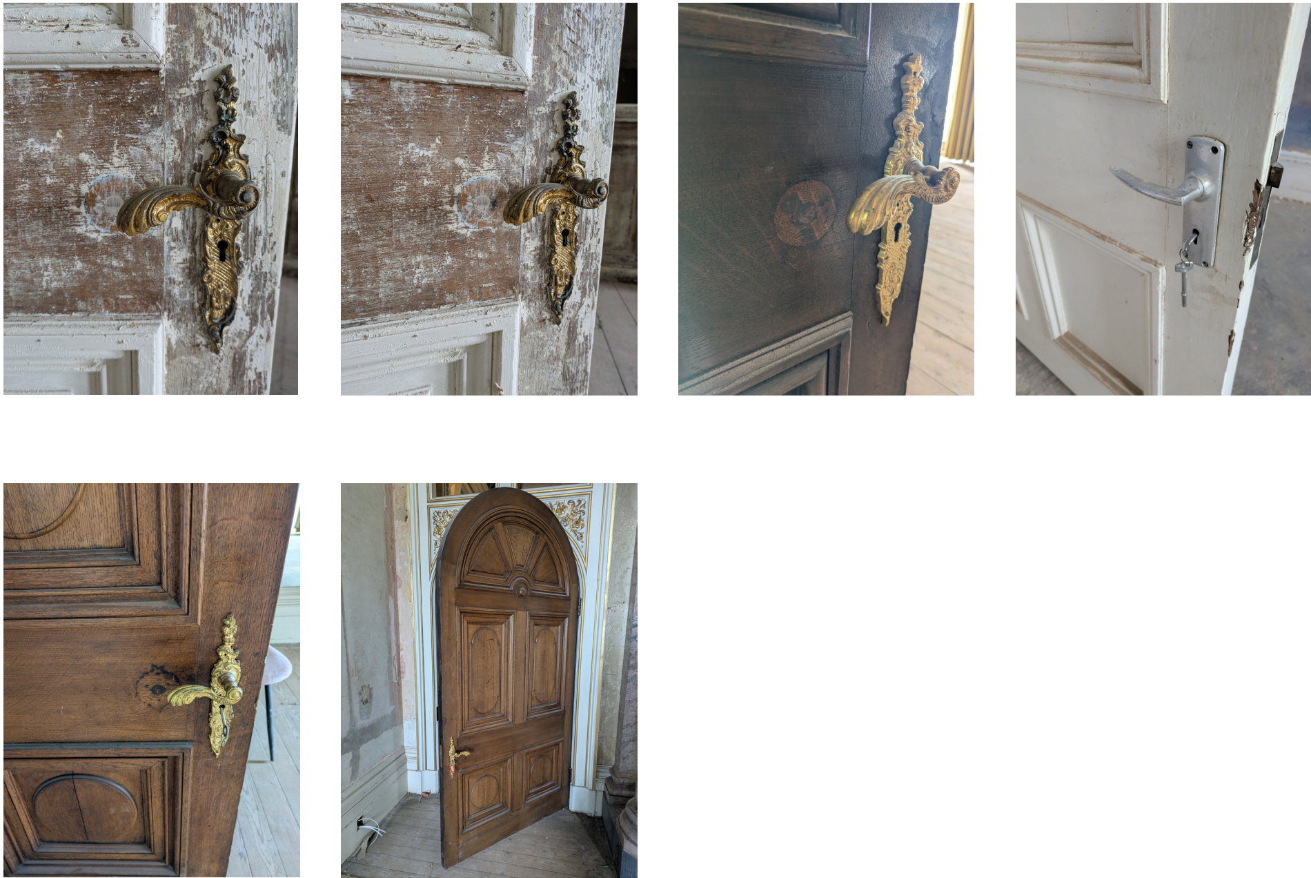
Examples of altered door handle and handle location
