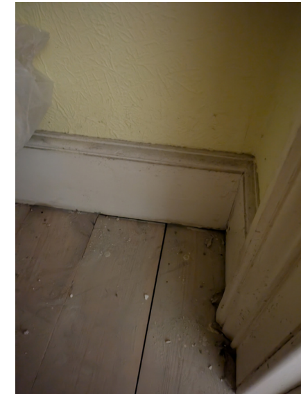
Original skirting to S18
