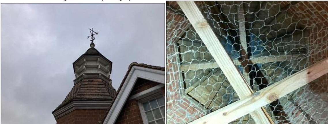
Photographs 9a(left) and 9b (right). 9a) exterior view of tower 2 taken from the northern aspect with view of the well-kept tiles noted across the feature. 9b) interior view of the tower from the base with view of the well-kept boarded roof and the wire mesh to centre of the image.
