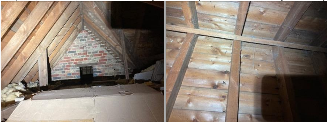
Photographs 6a (left) and 6b (right). 6a) View of the interior of void 2, facing east with view of the brick wall and the small opening into tower 1's void space. 6b) View of void 2's apex with view of the wooden board's tight seals and limited gaps which is consistent across the length of the void.
