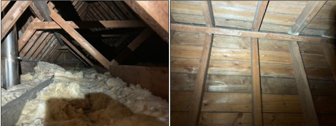
Photographs 4a (left) and 4b (right). 4a) View of loft void 1 from the void entrance with the image taken at the base with of the collar ties noted to the centre of image. 4b) View of void 1's apex with view of the wooden board's tight seals and limited gaps which is consistent across the length of the void.
