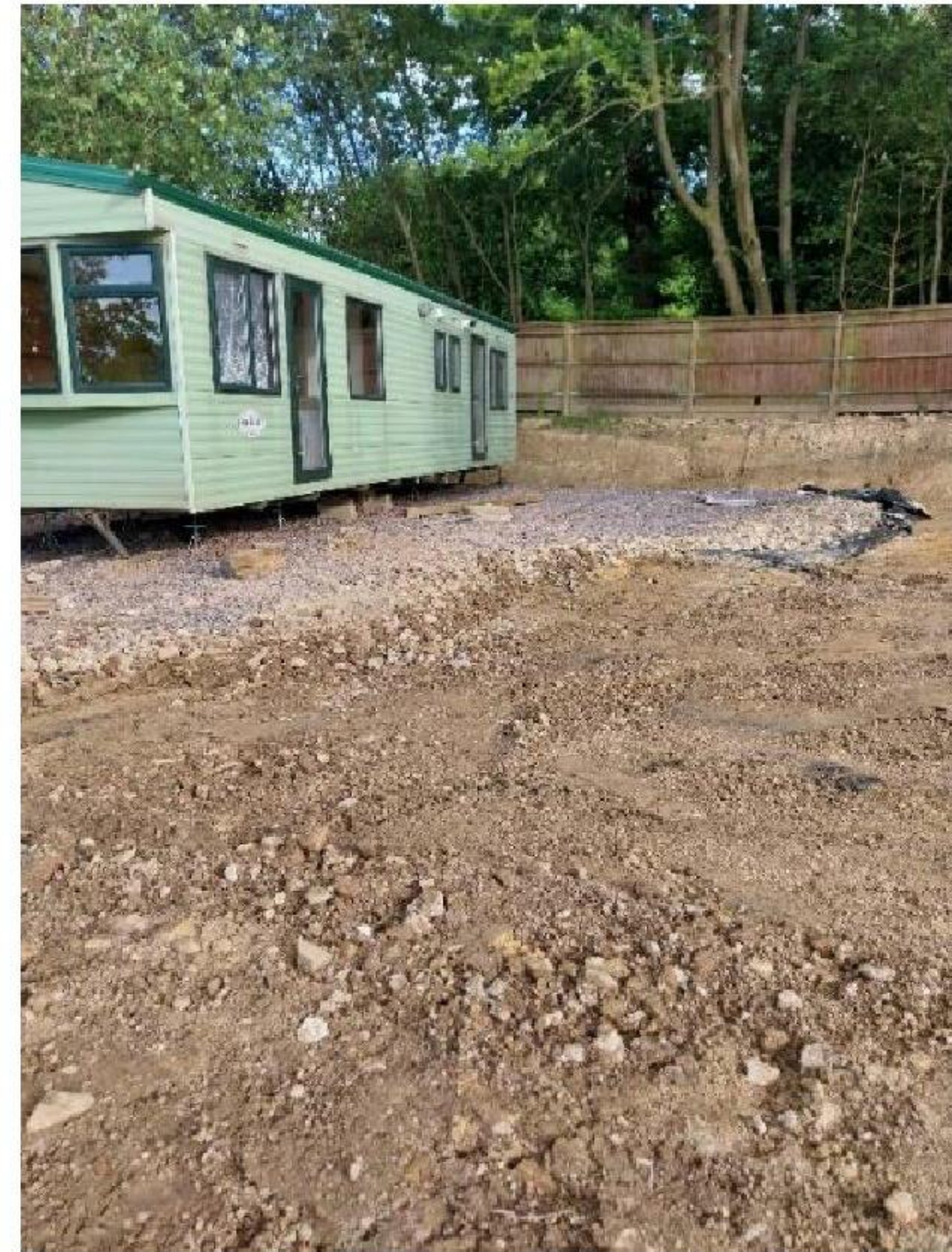
Figure 4 - North Western elevation of the mobile home
