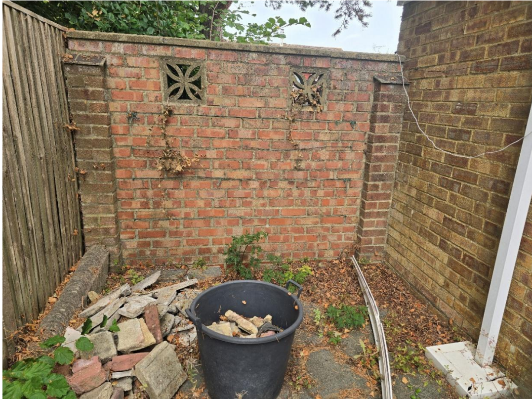
Photo 2 – Brick boundary wall reducing root growth to the rear of 17 combers
