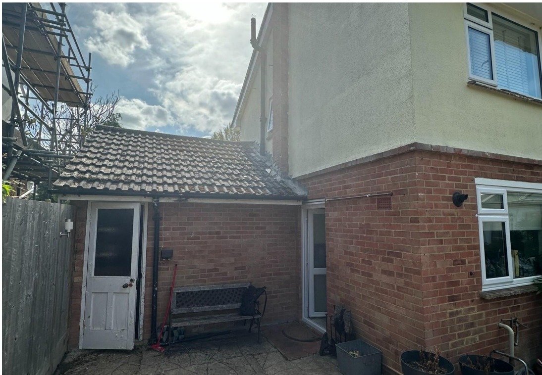
Figure 3 - Existing side/rear area behind the garage, within the area affected by the additional single-storey works.
