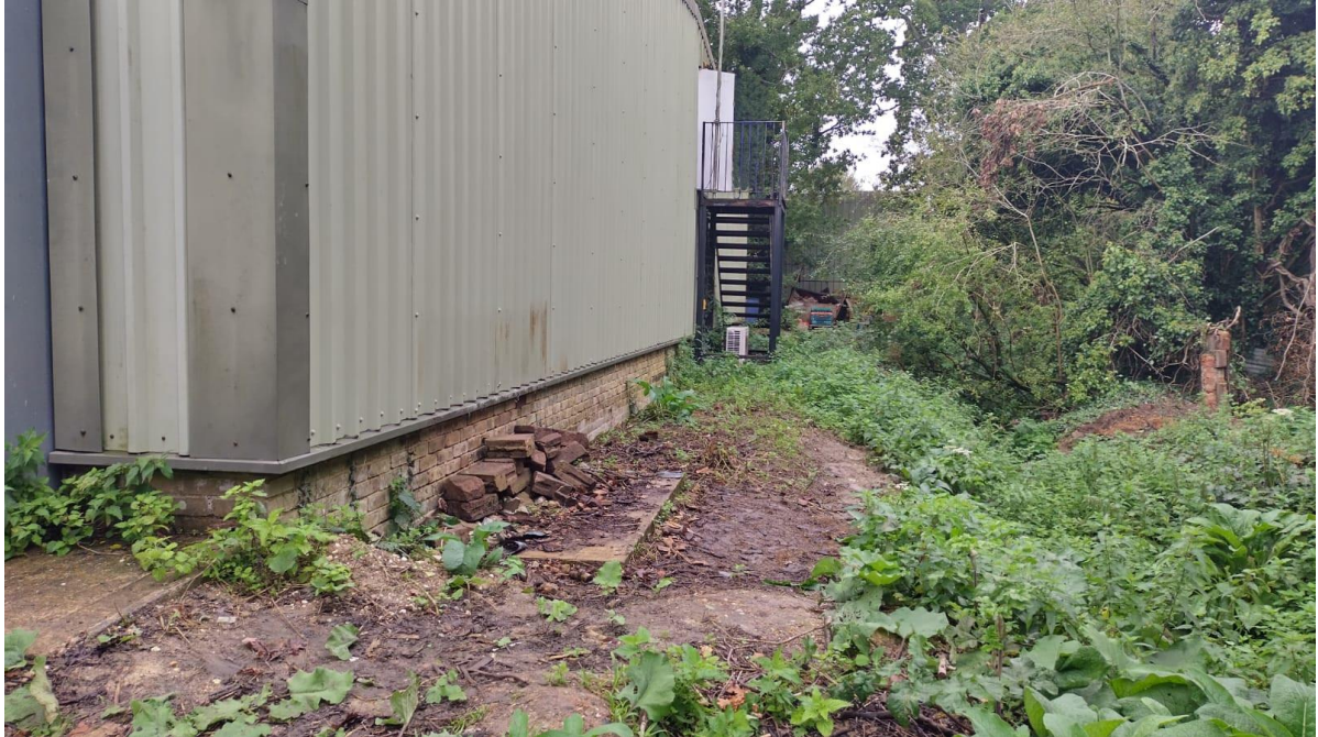
Figure 1: The application site, showing the rear elevation of Unit 19. The external staircase serves the adjoining unit.
