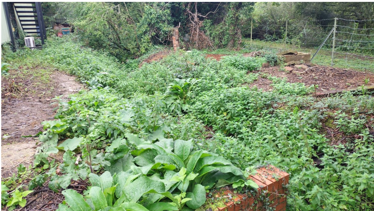
Figure 6: Vegetation, close up. The brick culvert is visible in the foreground
