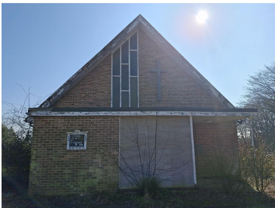
Figure 3: Exterior of the standing building
