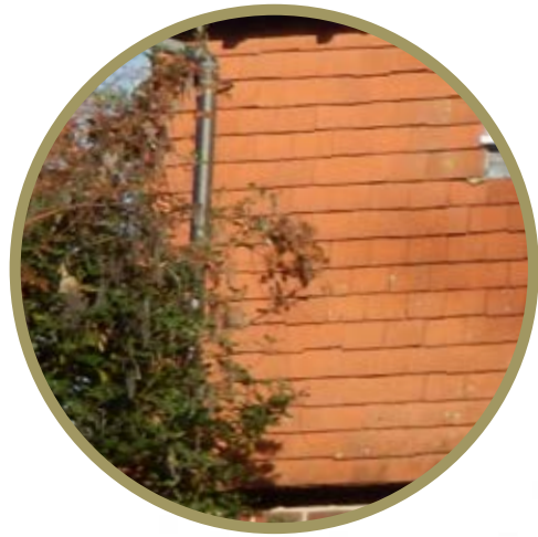
Tile hanging on upper floors of corner dwelling
