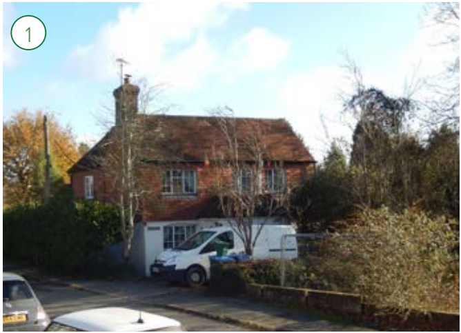
Cottage to the east of the site
