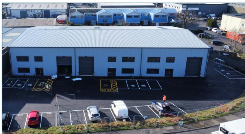
Photo of the recently completed unit
