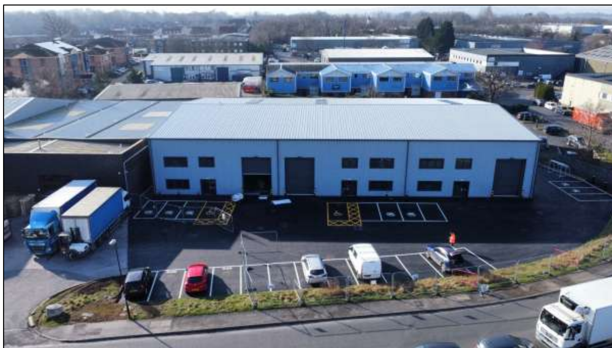
Figure 3. Photograph of Newly Constructed Site
