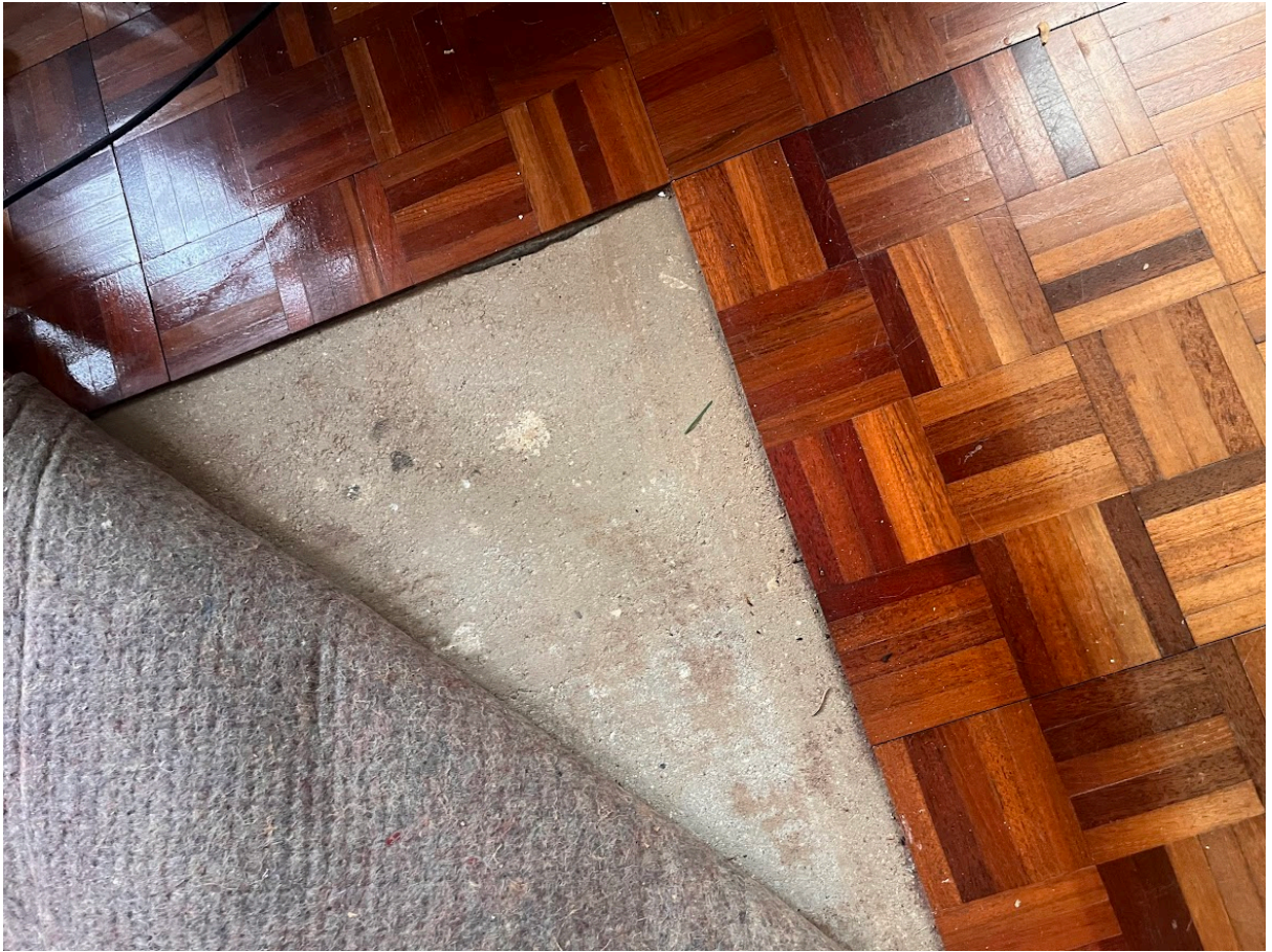
Parquet tiles and concrete floor
