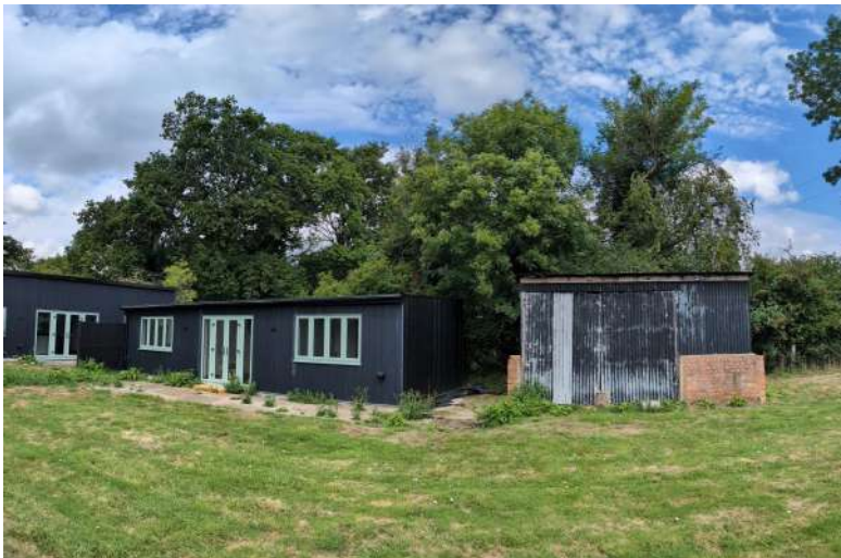
Photo 2: Trees to rear of existing structures.
