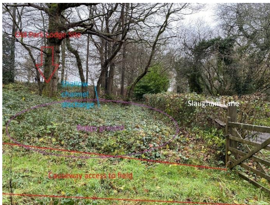
Photo 3 Existing Shallow Ditch outlet location (waterlogged ground)
