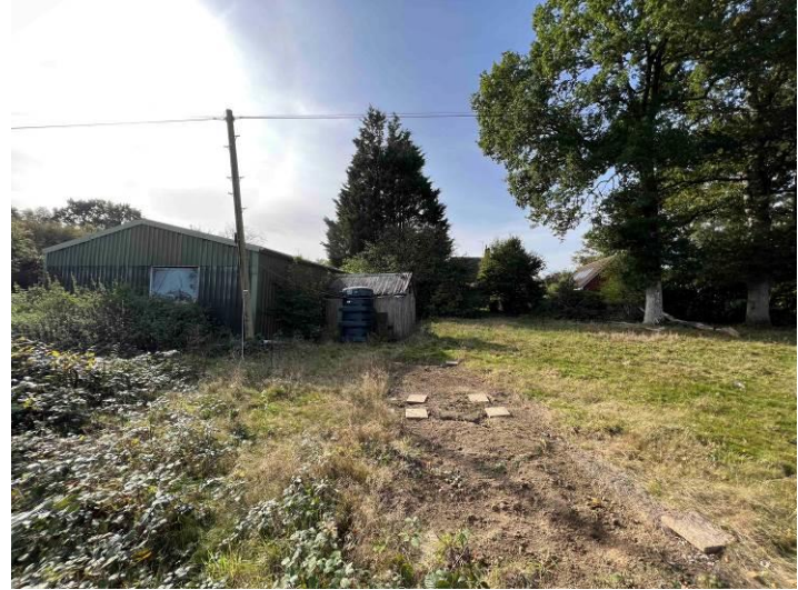
North elevation of barn (to be removed)
