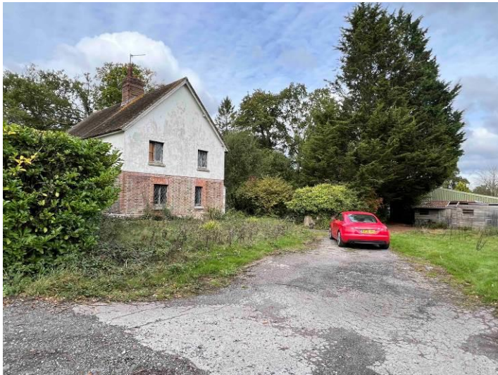
East elevation and site entrance
