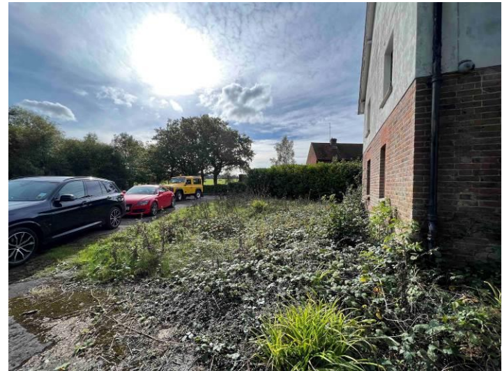
East elevation and driveway
