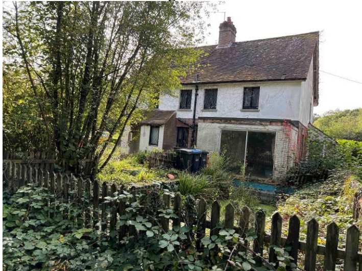
North (rear) elevation of existing property
