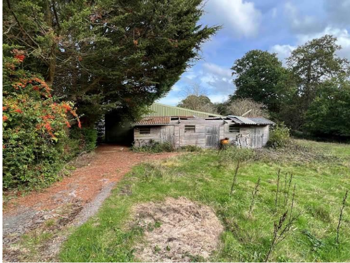
South elevation of barn and stable building
