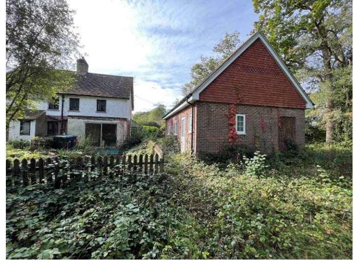
North elevation of house and garage
