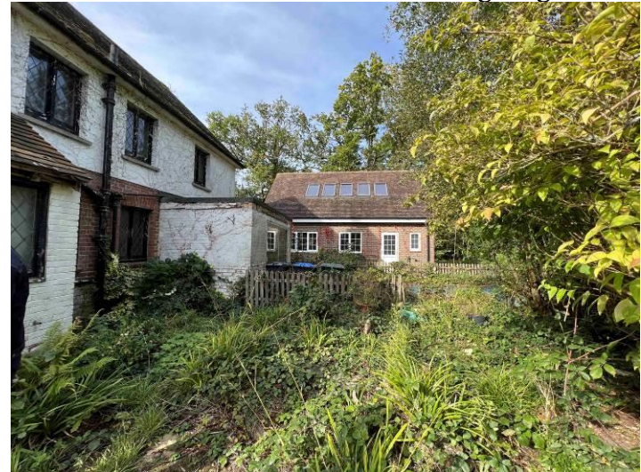
East elevation of garage (to be retained)
