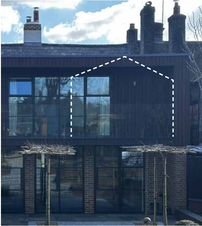
Recent photograph showing mass of historic outrigger visible through glazed openings - walls painted white
