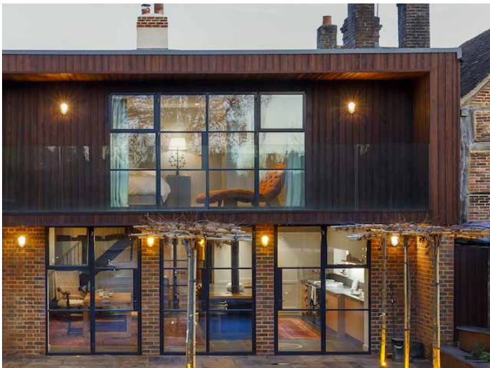
Recent photograph of rear elevation proving visibility of the gable through the new large windows to extension
