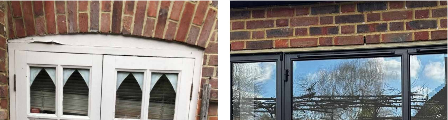
Comparison of brickwork used on the original (left) and re-constructed (right) bake house.
