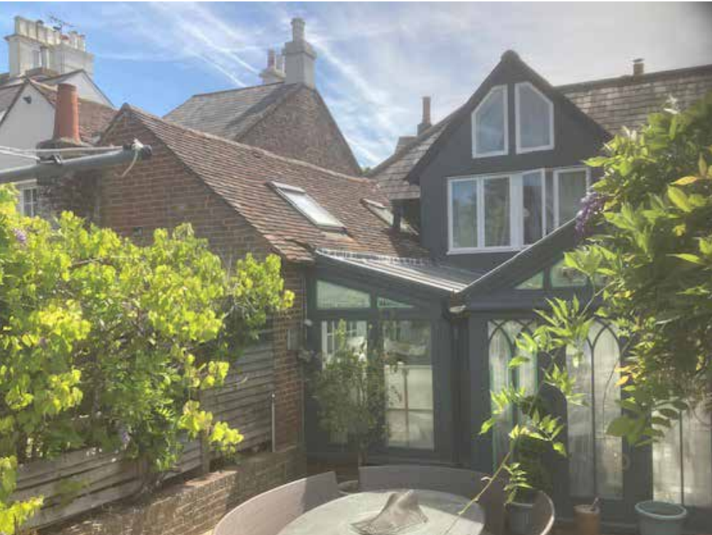
Rear view of Marlow House before works
