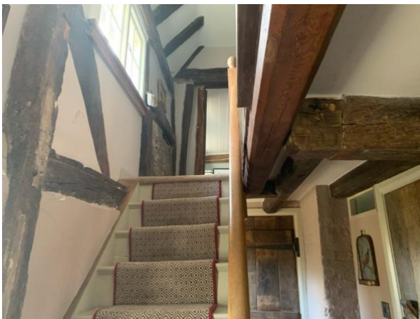
Service bay with modern staircase, truncated crossbeam C-C and joists with diagonal brace to post as opposed to a down brace. Note the split rail below the window. Also, the lower section of the post sees a filled in mortice where the crossbeam would have been tenoned into.
