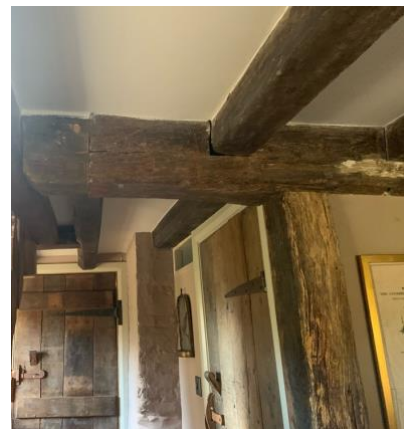
Service bay with modern staircase, truncated crossbeam C-C and joists with diagonal brace to post as opposed to a down brace. Note the split rail below the window. Also, the lower section of the post sees a filled in mortice where the crossbeam would have been tenoned into.
