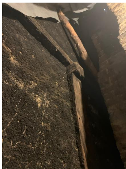
B-B South face Crown Post obscured. B-B North Face. The brick stack sits close Down braces are just visible. to the soot blackened daub and collar.
