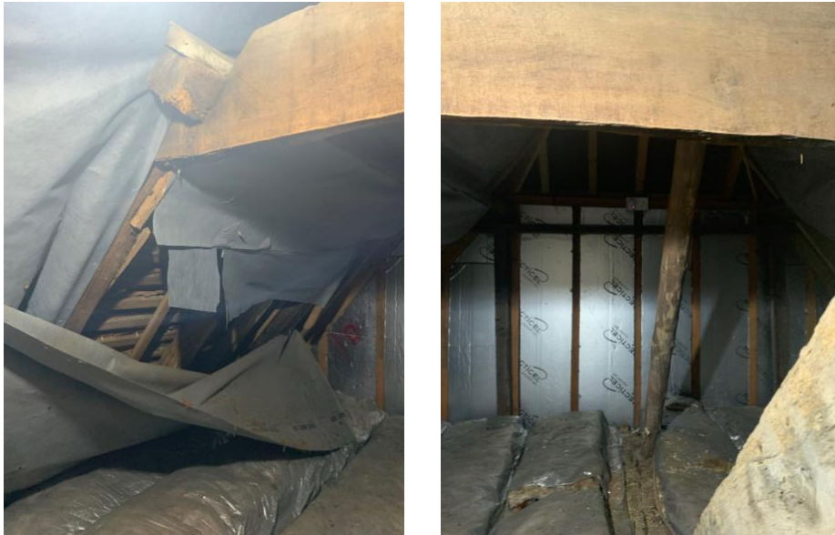
Collar clasp side purlin (truncated) above service chamber. Evidence of Victorian and 20 th century timbers. Note the bark stripped branch acting as a supporting rake.
