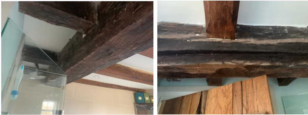
Continuation of crossbeam C-C through partition to west side of gf bathroom. Evidence of former door from hall passage.
