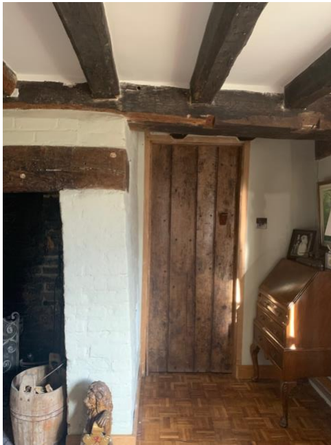
Baffle entry created by introduction of inglenook but later relocated to the service bay.
