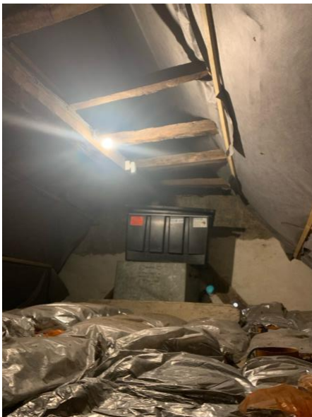
B-B South face Crown Post obscured. B-B North Face. The brick stack sits close Down braces are just visible. to the soot blackened daub and collar.
