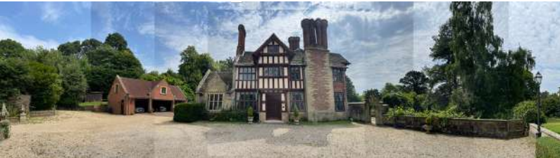
V1 Chownes Mead Listed Building and Garage (NW)
