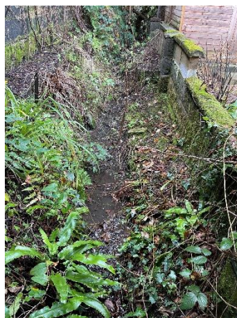
Fig 02 – the main body of the ditch
