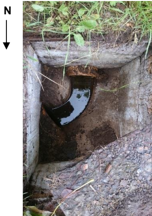
Manhole Open Photo
