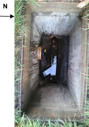
Manhole Open Photo
