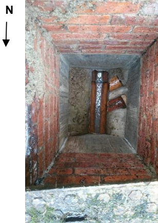
Manhole Open Photo
