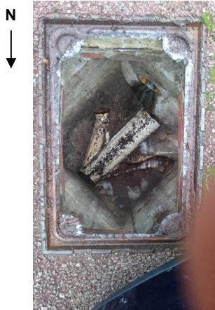
Manhole Open Photo
