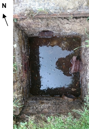
Manhole Open Photo
