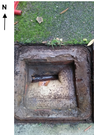
Manhole Open Photo
