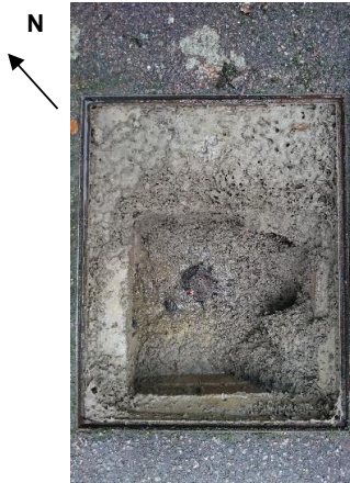
Manhole Open Photo
