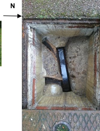
Manhole Open Photo
