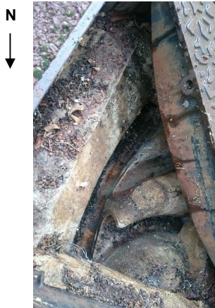
Manhole Open Photo
