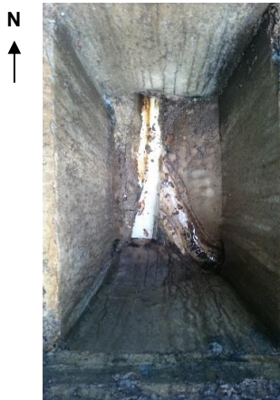
Manhole Open Photo
