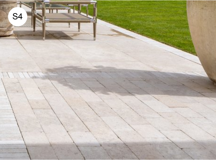
Block Pavers providing textural contrast
