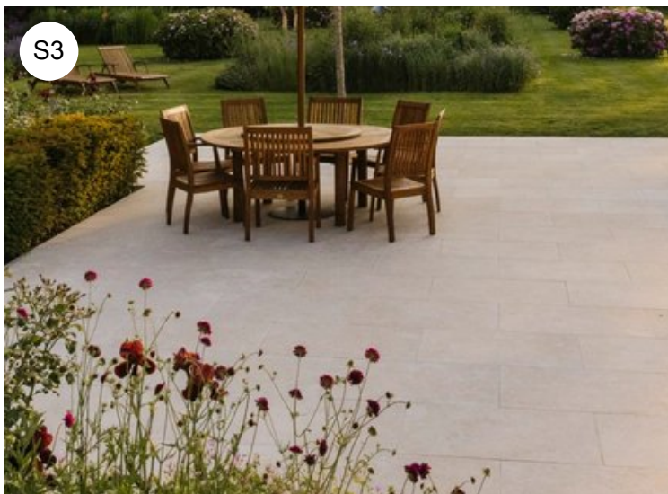
Honed Natural stone paving around Main House
