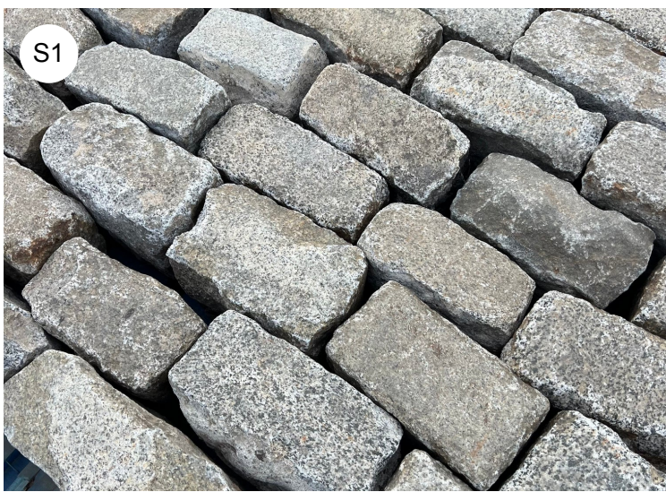
Reclaimed cobbles rumble strips
